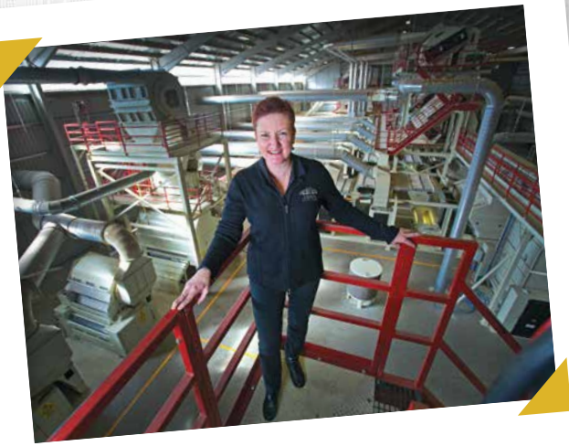
The $25 million Southern Cotton gin was built in under 12 months.
