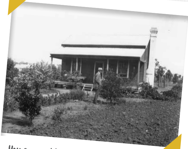
You can visit Henry Lawson's restored cottage at Farm 418, Naalbata Road Leeton NSW.
