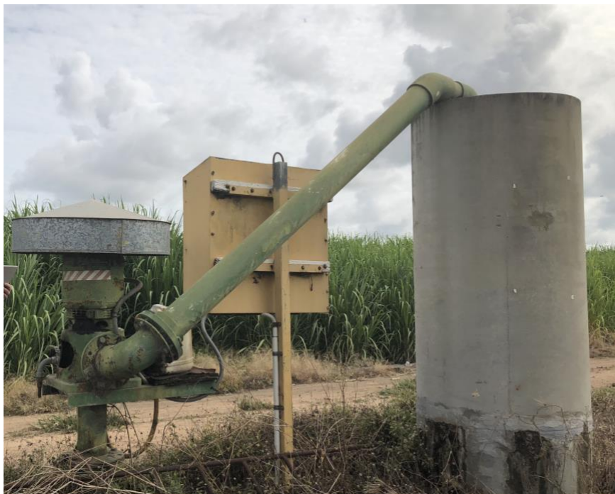
Figure 11: A grid-connected stationary pump at Wilmar farms, Ayr.
