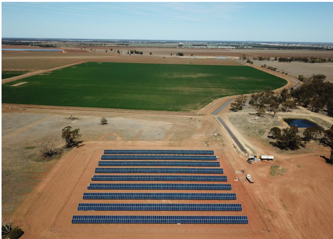
Figure 9: 500kW solar system on a farm near Narromine, NSW (Photo source: ReAqua)
