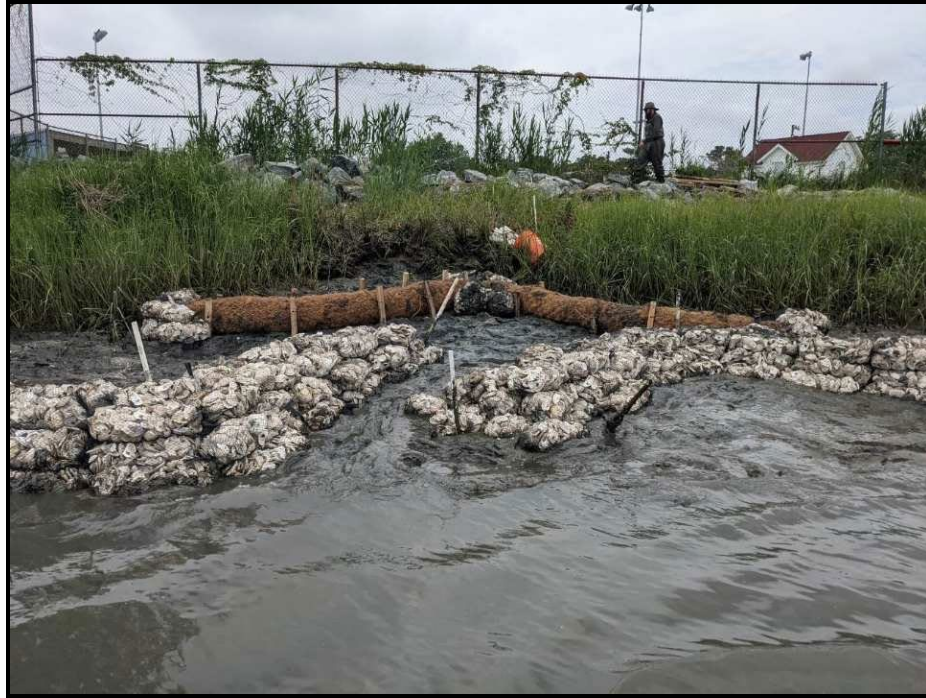
Figure 7. Oyster shell bags placed in a curved overlapping formation allowing living resources and hydrologic exchange (Photo Credit: DNREC Wetland Monitoring and Assessment Program).
