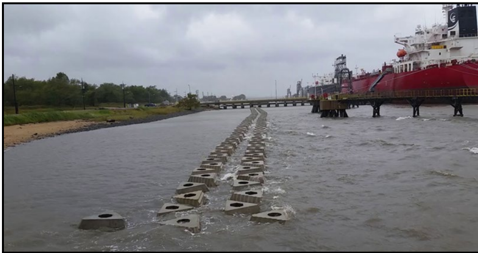
Figure 1. Wave Attenuation Devices® (WADs®) dissipating wave energy while also providing interstitial space for habitat (Photo Credit: Chris Pfeifer).
