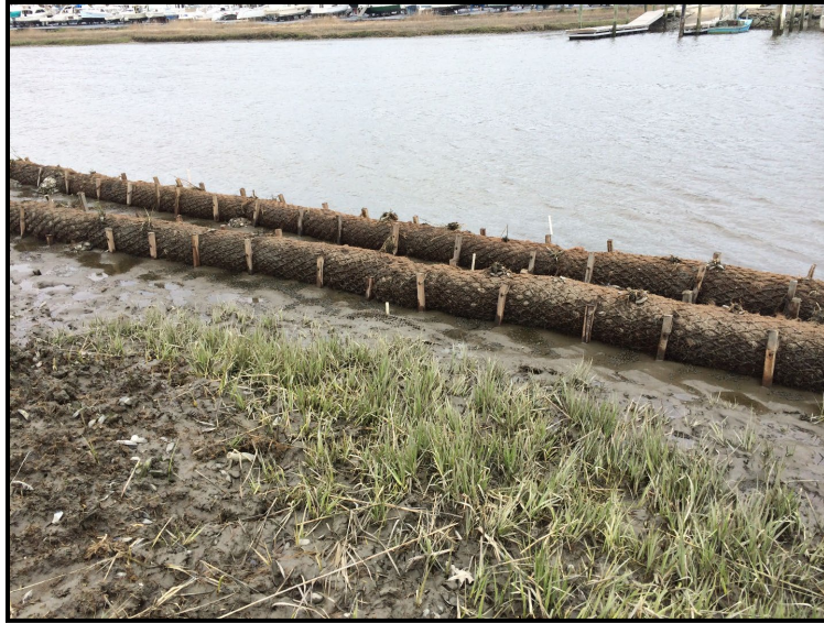
Figure 5. Newly installed coir fiber log terraces awaiting natural sedimentation (Photo credit: DNREC Wetland Monitoring and Assessment Program).
