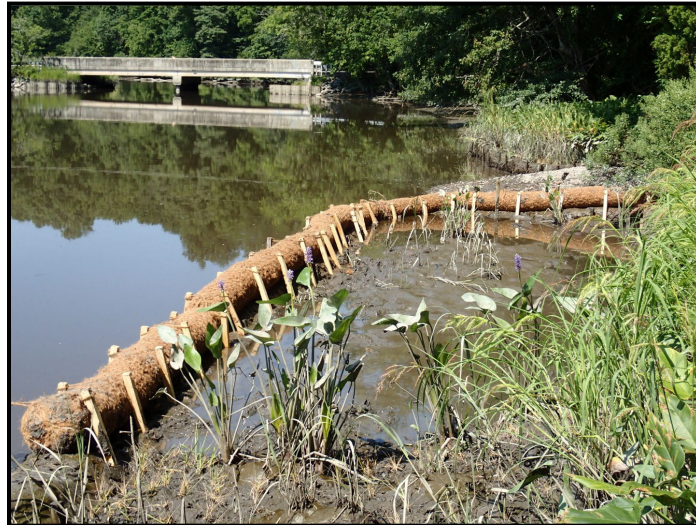
Figure 8. Wood stakes and twine installed to anchor coir logs (Photo credit: DNREC Wetland Monitoring and Assessment Program).
