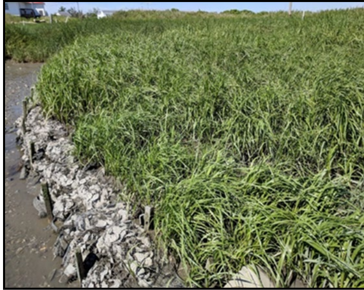
Figure 2. Oyster Shell bag base-stabilization (Photo Credit: Partnership for the Delaware Estuary).
