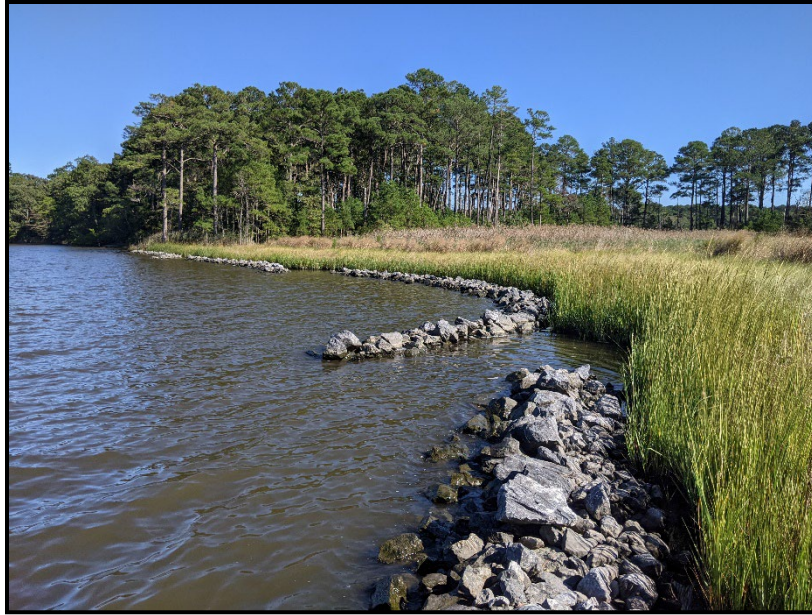
Figure 10. Rock toe sill reducing wave energy (Photo Credit: Chris Pfeifer).
