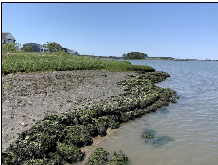
Figure 9. Oyster shell bags tightly stacked forming a toe (Photo Credit: Douglas Janiec).
