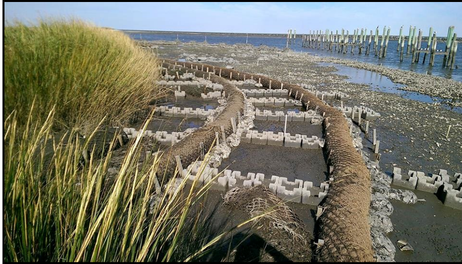
Figure 4. Oyster Castle® groin placed inside and along the front of a living shoreline (Photo Credit: Partnership for the Delaware Estuary).
