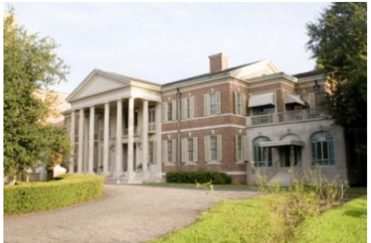
The Phelan Mansion, Beaumont, TX. Photo: Courtesy of Marsh Waterproofing, Inc.
