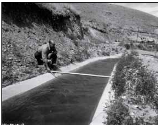
Showing streamflow in a cemented ditch. Hanson - Boyle Ditch, circa 1960. Teton Conservation District archives.
