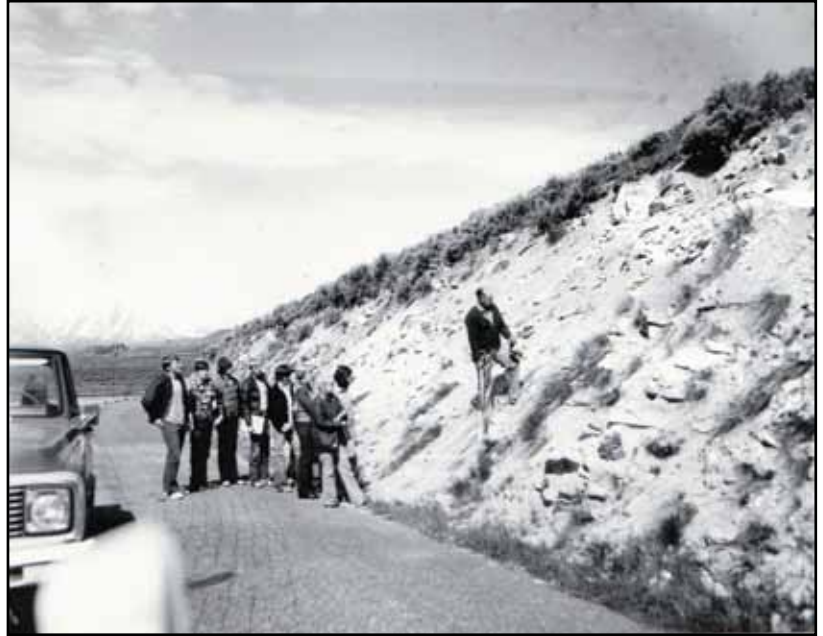
Don Lewis, soil scientist, explains the limitations of a shallow site during a 4-H conservation camp. Photo by Jim Rowles, circa 1975. Teton Conservation District archives.
