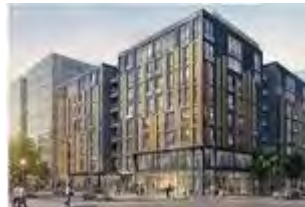
The Elle Apartments 1111 20th St NW (161 Units)
