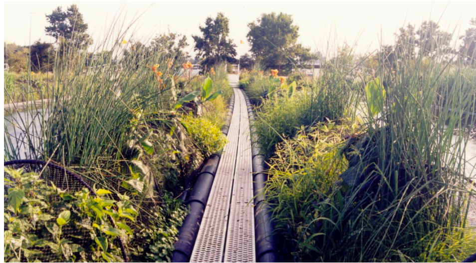
For an area of 2 acres, a Aquatic Restorer installed for Tyson's poultry processing facility in Berlin, Maryland typical installation can have 3-4 units depending on how quickly the client wants to digest the sediment. The largest installation of the Aquatic Restorer for lagoon treatment to date processes 1 million gallons per day. Photo © John Todd Ecological Design
