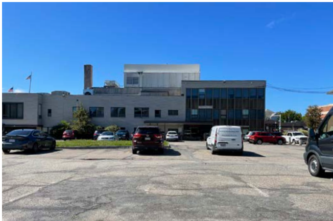
Left: Any development of the municipal parking lots would be by-right with site plan review.
