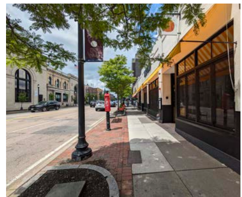
The Plan provides on-street parking along key retail frontages adjacent to the Square, including Main Street (shown here), Pleasant Street, Mount Auburn Street, and Arsenal Street / North Beacon Street.
