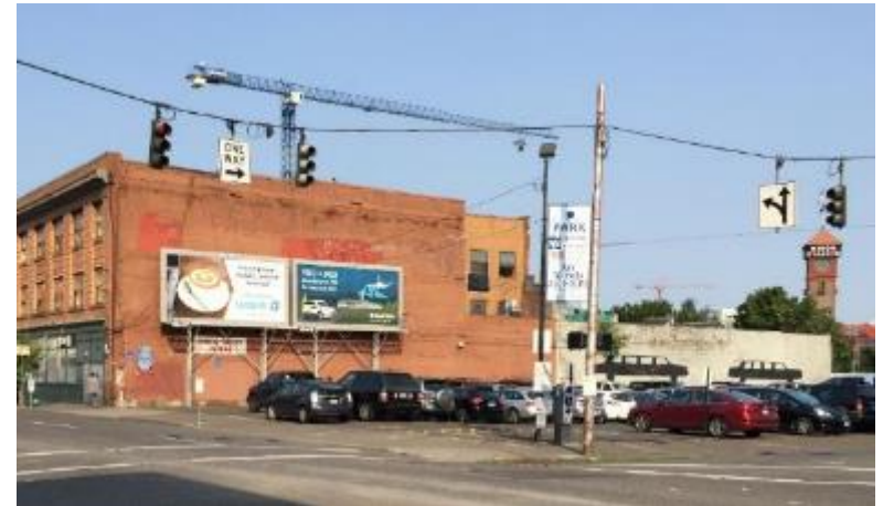
Surface parking lots and underutilized parcels contribute to an austere pedestrian environment along NW Glisan St. between NW Broadway and the Steel Bridge
