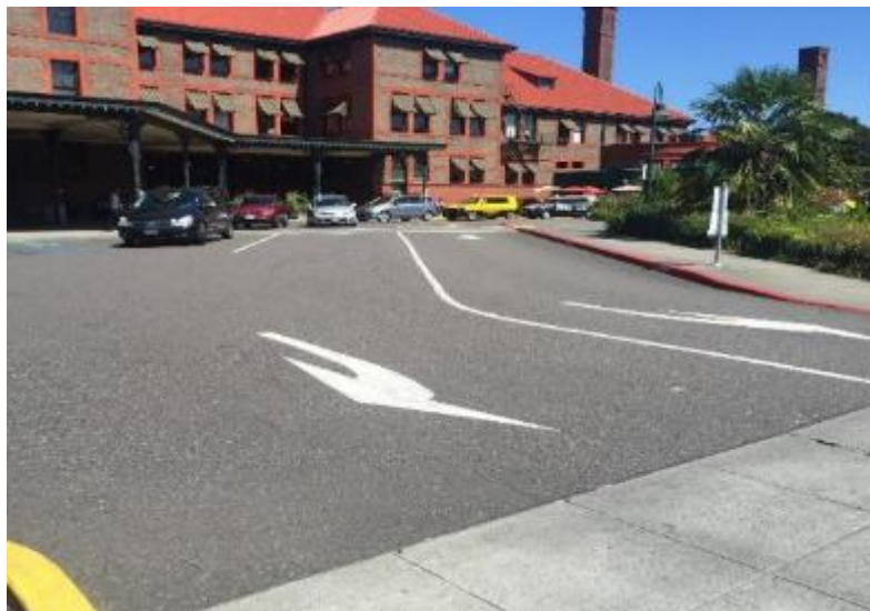
Buses sometimes enter the driveway exit in the opposite direction to avoid driveway congestion
