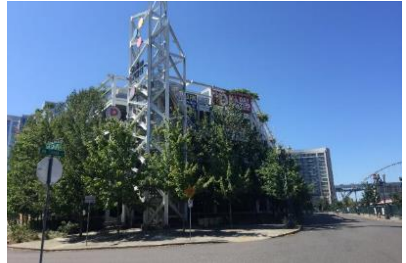
Station Place garage with hourly, daily, and overnight parking
