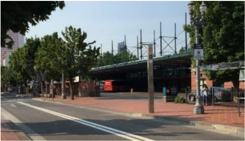
Curb cuts provide access to off-street bus facilities at Union Station, the TriMet layover facility, and the Greyhound Terminal (shown); however these driveways also interrupt the street wall and create mid-block pedestrian conflicts.
