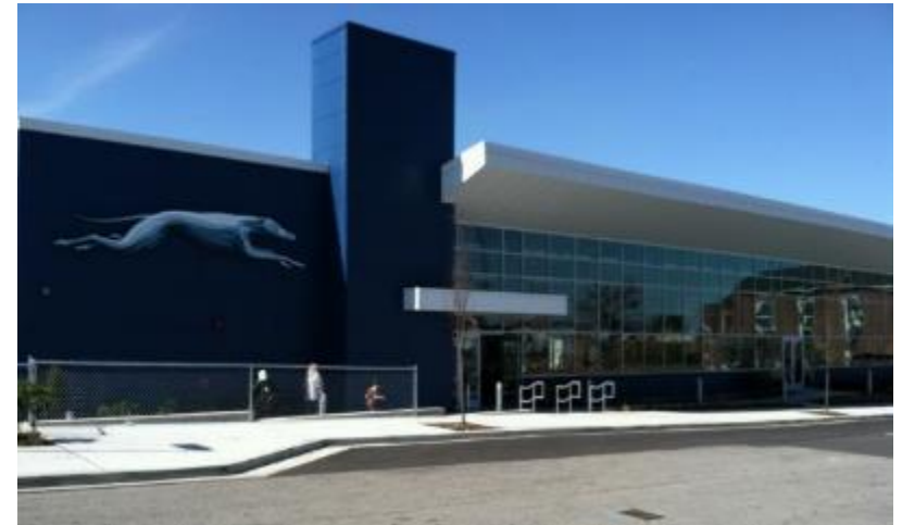
Nashville Greyhound Terminal – Relocated to a former car dealership site to accommodate the Music City Center redevelopment project. Nashville, TN
