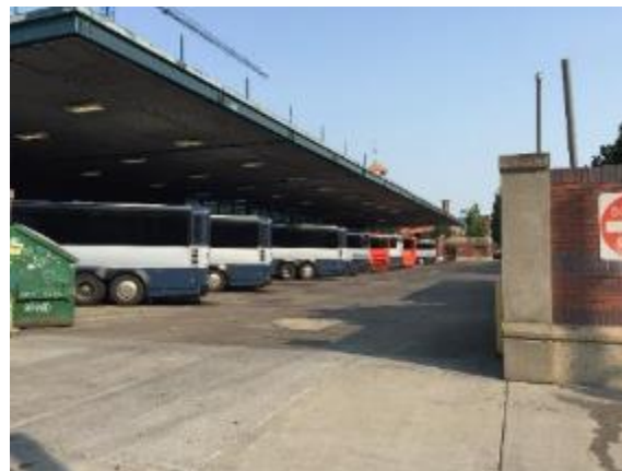
Greyhound Terminal vehicle egress (along NW Glisan St. between NW 5 th and 6 th Avenues) provides an inactive edge and pedestrian-vehicle conflicts at the curb cut.
