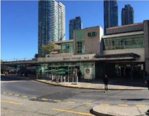
Union Station Bus Terminal (GO Transit) Toronto, ON
