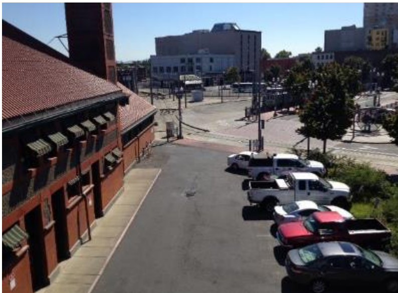
Amtrak employee parking near Union Station Annex – proposed for removal to create Annex Plaza
