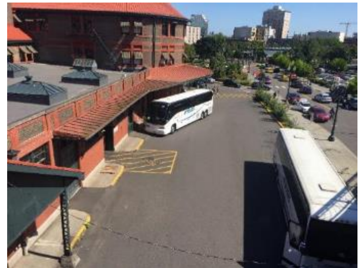
Union Station bus loading and layover area
