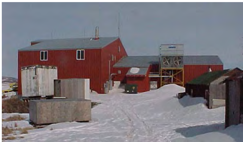
Unalakleet Fish Processing Plant in April, 2000. The main processing area is in the tall part of the building.
