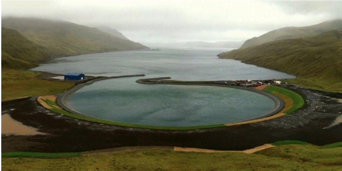
Figure 3: Akutan Harbor construction in progress Source: https://akutanharbor.com/
