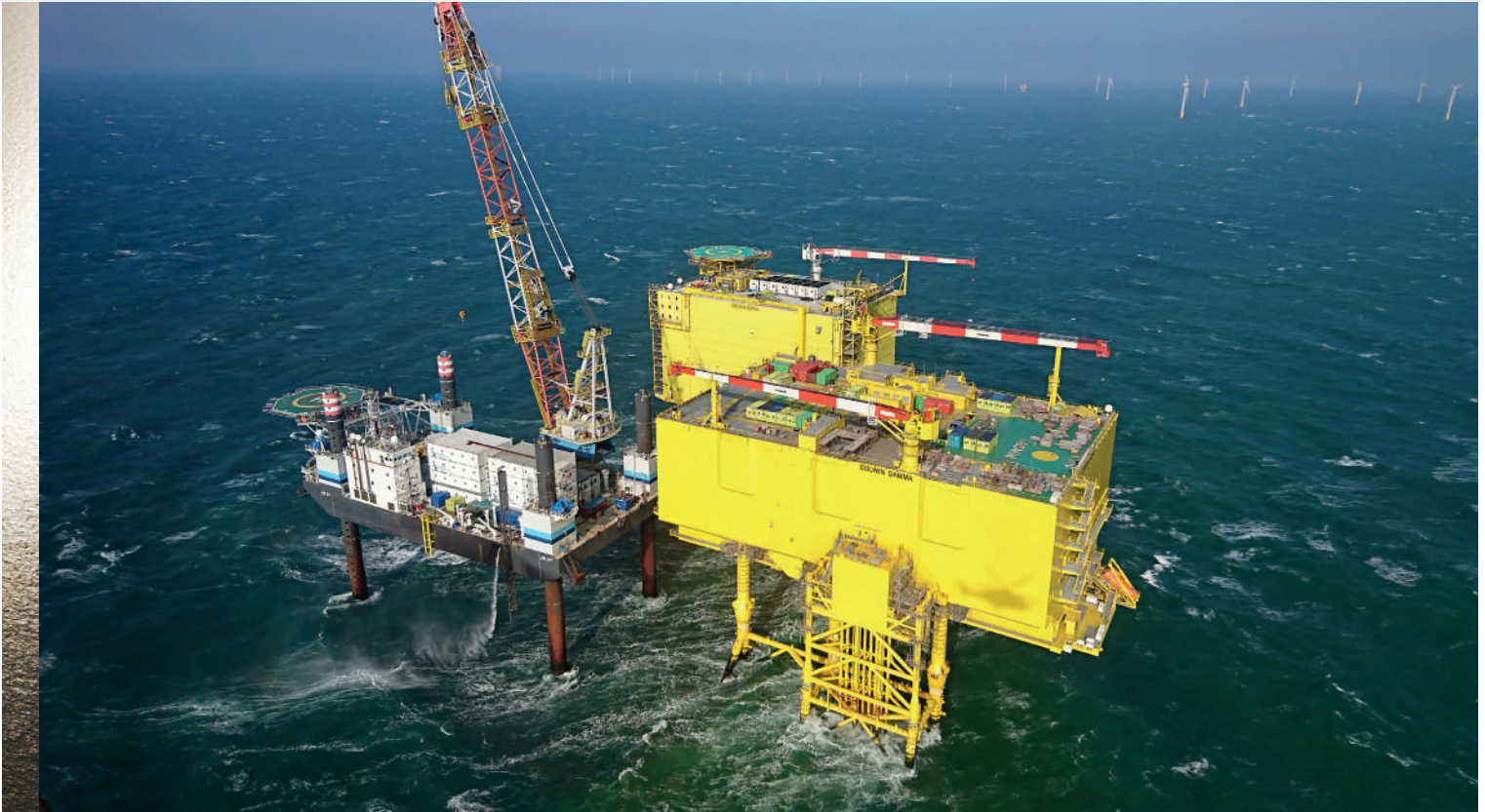
Picture: Dolwin3 (CIP project)
