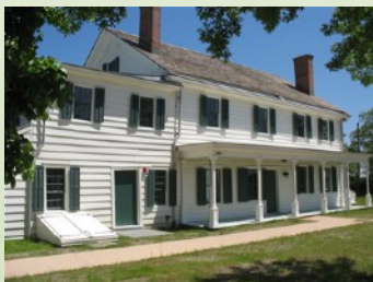
Bayshore Waterfront Park Activity Center (Seabrook-Wilson House)
