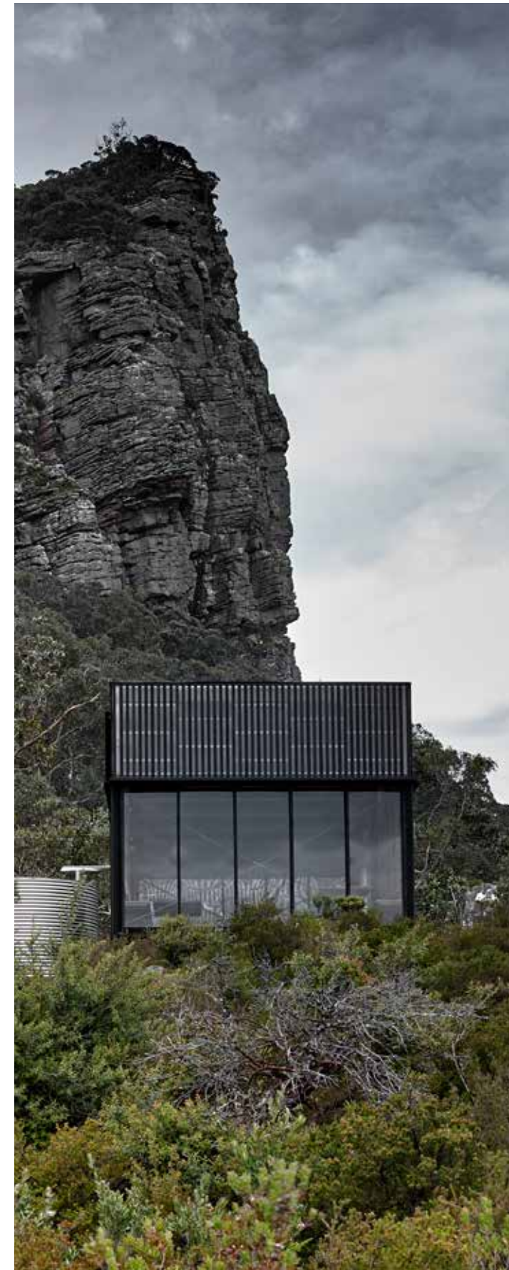
The communal hut at Mud-Dadjug (Mt Abrupt). opposite top The communal shelter at Stony Creek Group Campground. Photography: Shannon McGrath. bottom left Trekking along the main range from Briggs Bluff. right Tent pads and communal shelter at Djardji-djawara. Photography: Shannon McGrath
