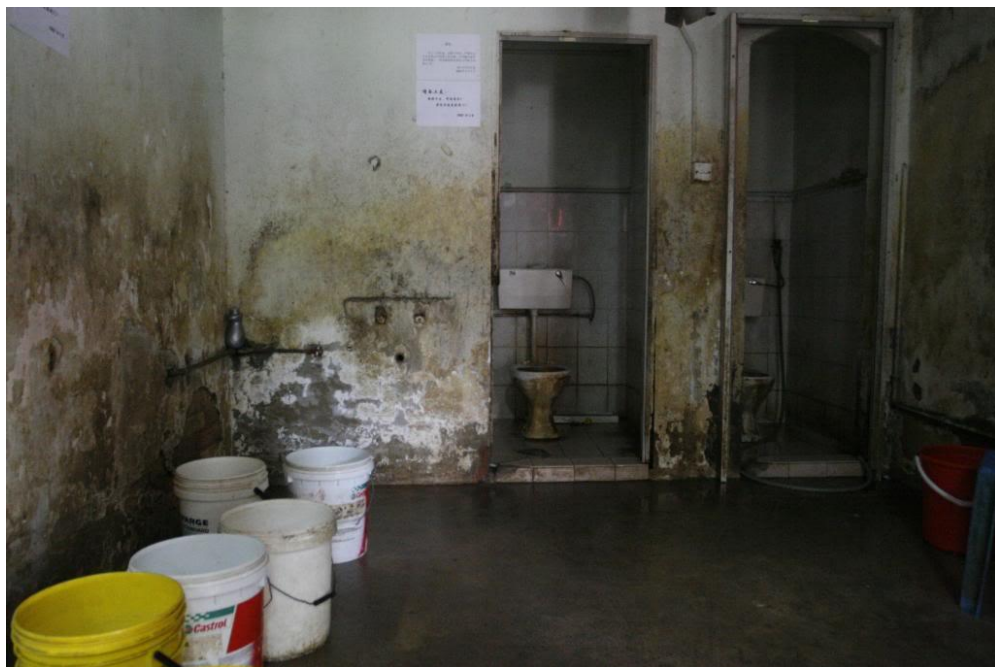
Toilet and bathing facilities Photo credit: Stephanie Chok
