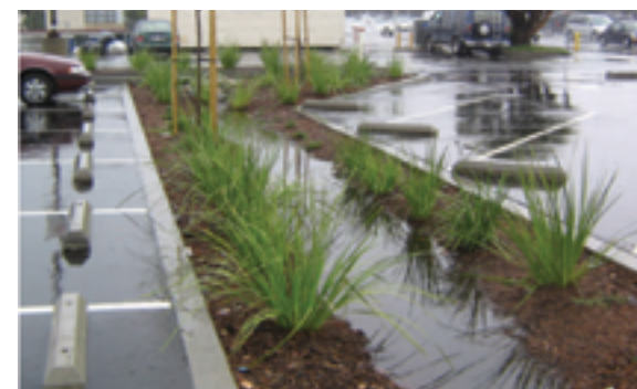
Low-impact development and green infrastructure as featured in the 2010 Groundwater Augmentation Study
