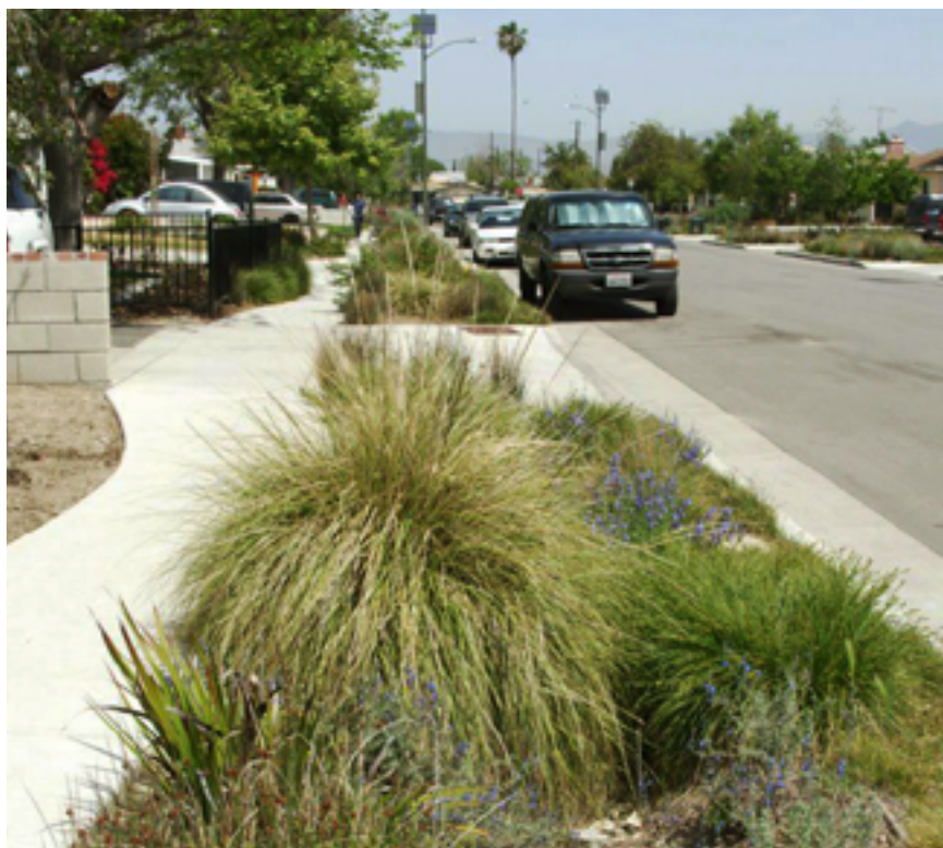
The Elmer Avenue retrofit was completed in 2010. Perforated pipeline to capture grey water was added beneath the street. New sidewalks, curbs and bioswales were added.
