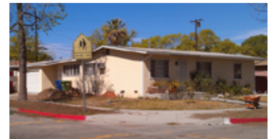
Fernandez residence prior to retrofit
