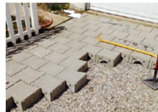
Permeable driveway in progress
