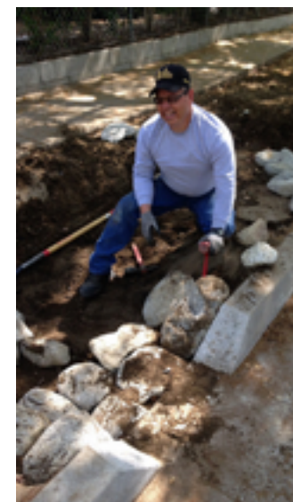
Parkway retrofit in progress
