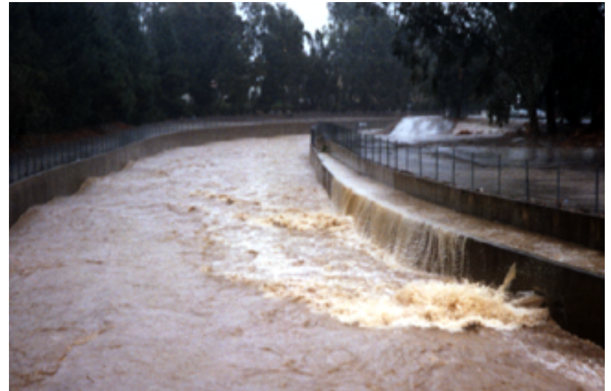
Concrete flood control channels direct stormwater to the Pacific Ocean.
