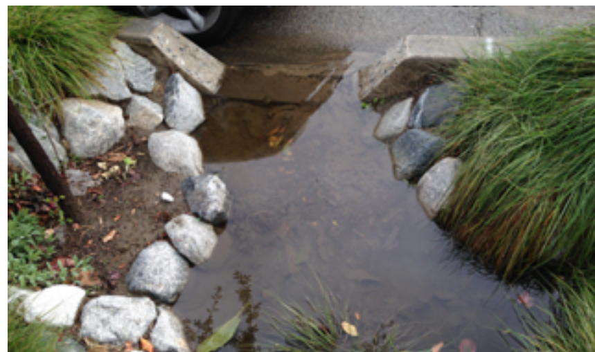
Water LA is working with the city’s Bureau of Sanitation and Bureau of Engineering to adopt standard plans for Water LA strategies such as parkway retrofits with curb cuts.
