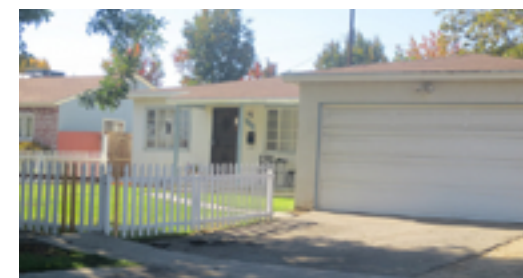
Hopkins residence prior to retrofit
