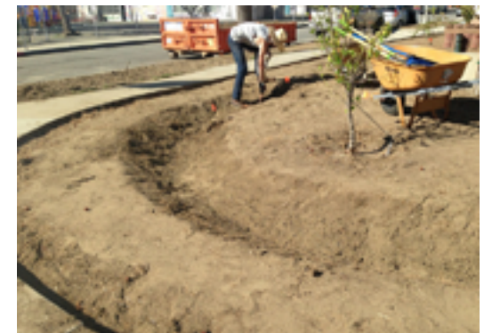
Rain grading in progress
