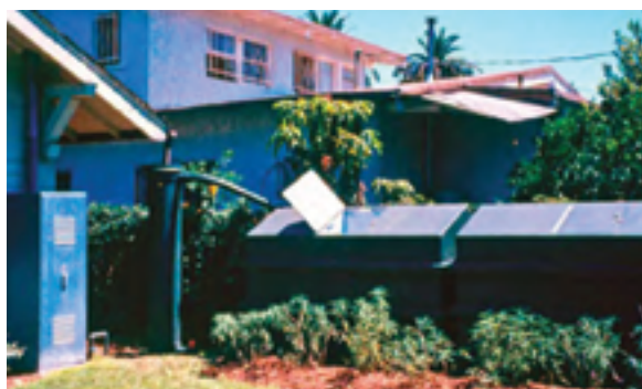
The “Hall House” included a cistern system, capturing stormwater from the roof.
