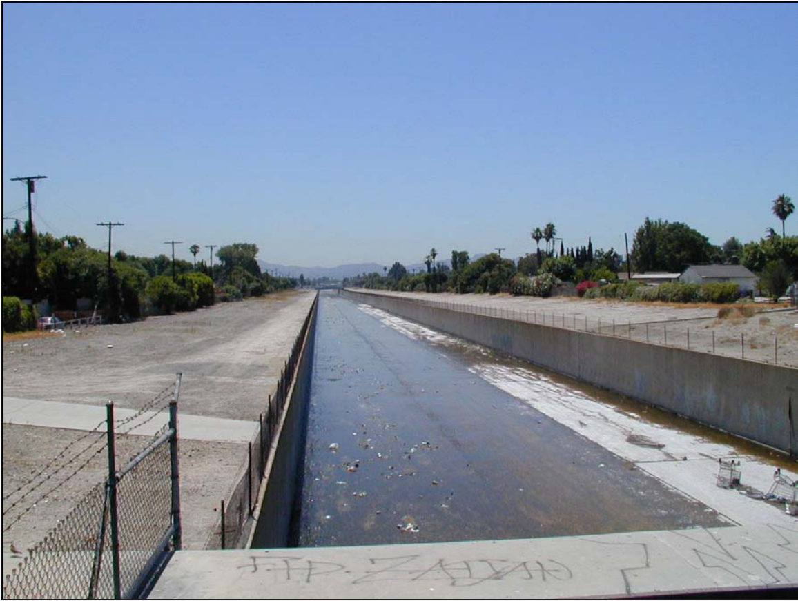
Figure 4 Existing Conditions below Pacoima Wash
