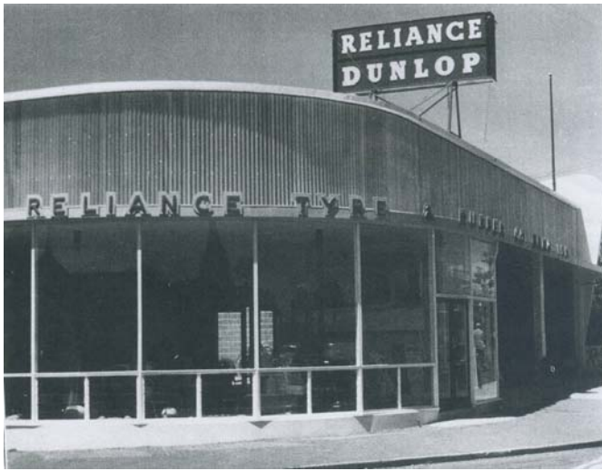
Reliance Tyre and Rubber Co building, 1955, D.A Wilson Architect. Clark J and Walker P, Looking for the Local p150
