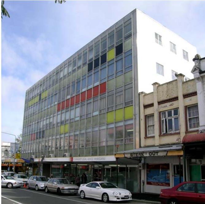
Government Life Building from Guyton Street 2007. Photograph by Author.
