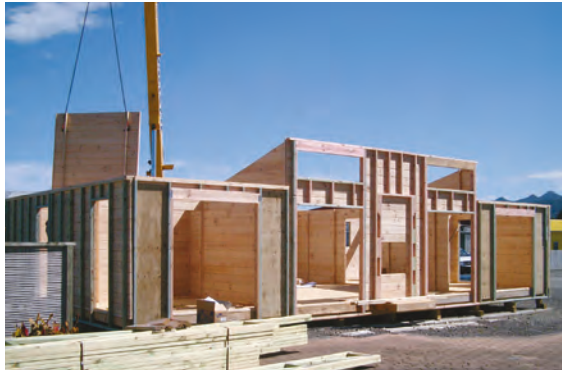
Timber panels assembled as house structure.
