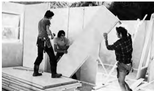
Light Modular Construction panel assembly.
