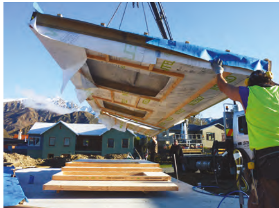
Custom panel assembly at site.
