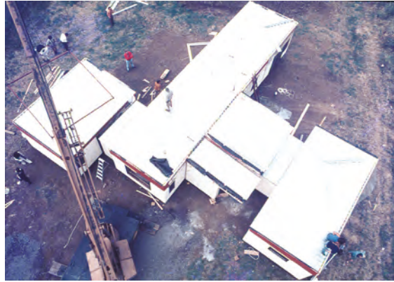
Aerial view of house on site.
