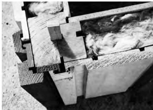
Light Modular Construction panel corner joint detail.
