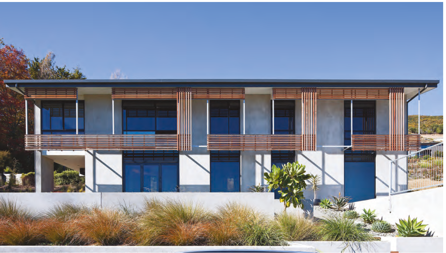
Tilt Panel House Tasman Bay.
