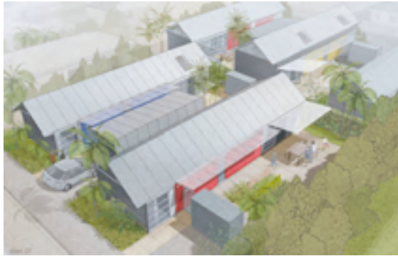
Competition entry by Geoff Fletcher Architects for Starter Home competition 2009 using metal SIPs panels as roofing.
