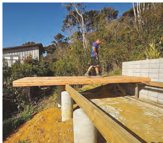
Cantilevered CLT floor panels.
