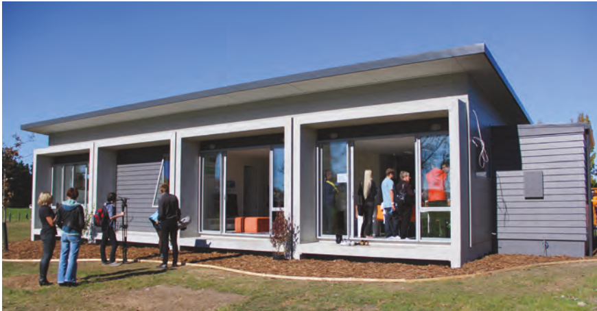
Precast concrete Falcon Rakaia House.
