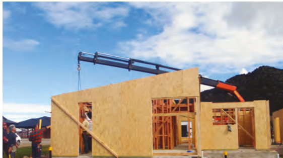
Building a High Performance House using SIPs.
