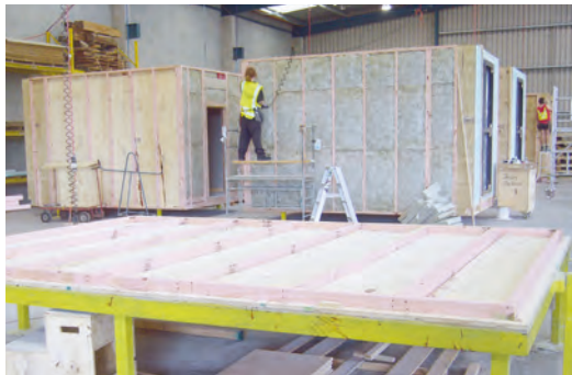
Modules manufactured in Stanley's Matamata factory.
