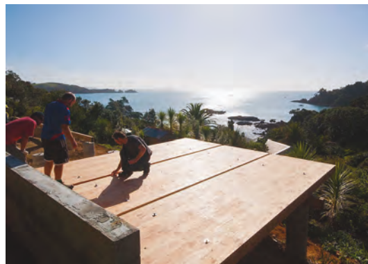
CLT floor panels create an immediate working platform.
