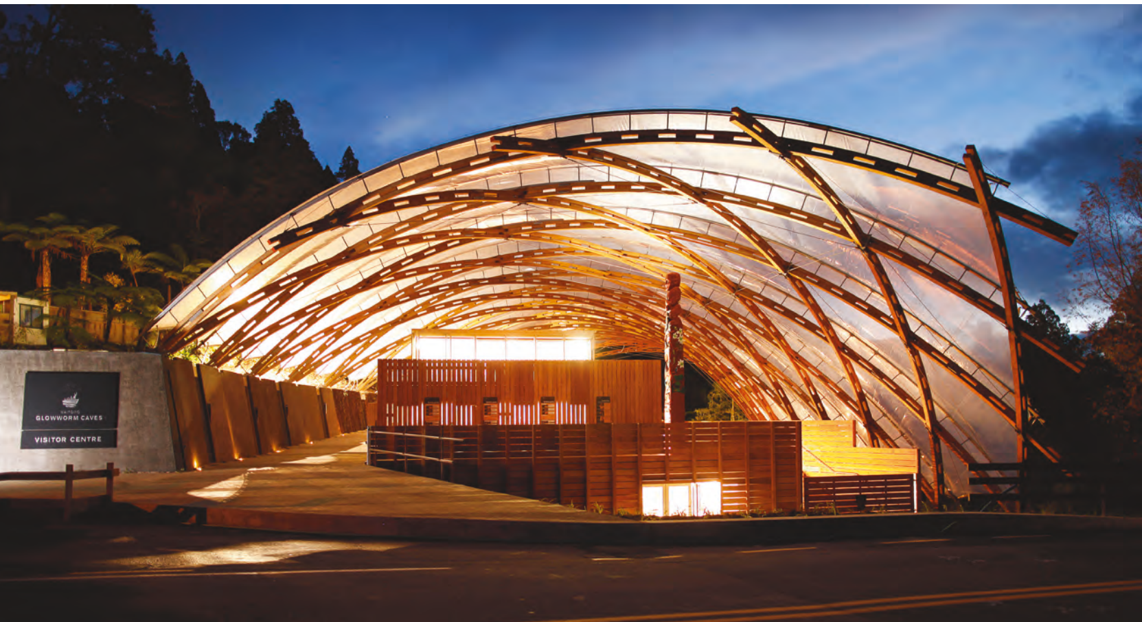
The Waitomo Caves Visitor centre with LVL interwoven I beams detail below.
