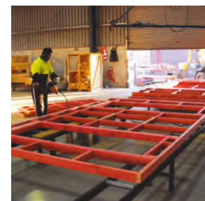
Component-based pre-nailed roof truss and wall frames.
