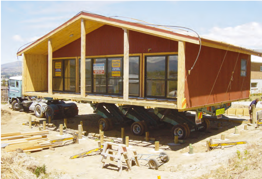
Alpinehaus dwelling being positioned for lowering at site.
