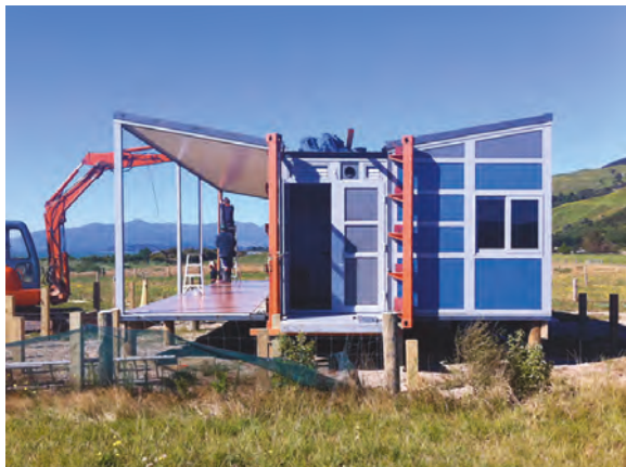
Habode being unfolded at the final site.
