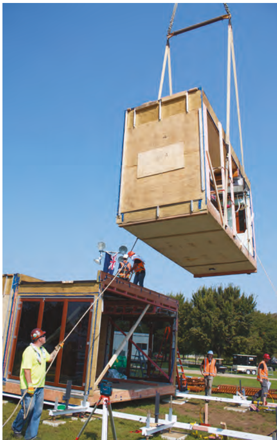
Modular volumes being set into position on site.
