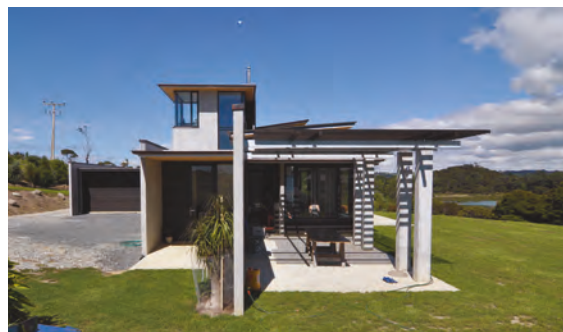
Precast concrete panels assembled in residential construction.
