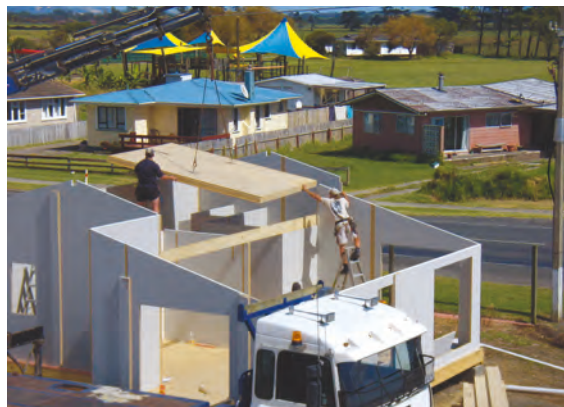
Triboard House assembly: stressed-skin floor panels, Triboard exterior and interior wall panels, stressed-skin ceiling and roof panels.
