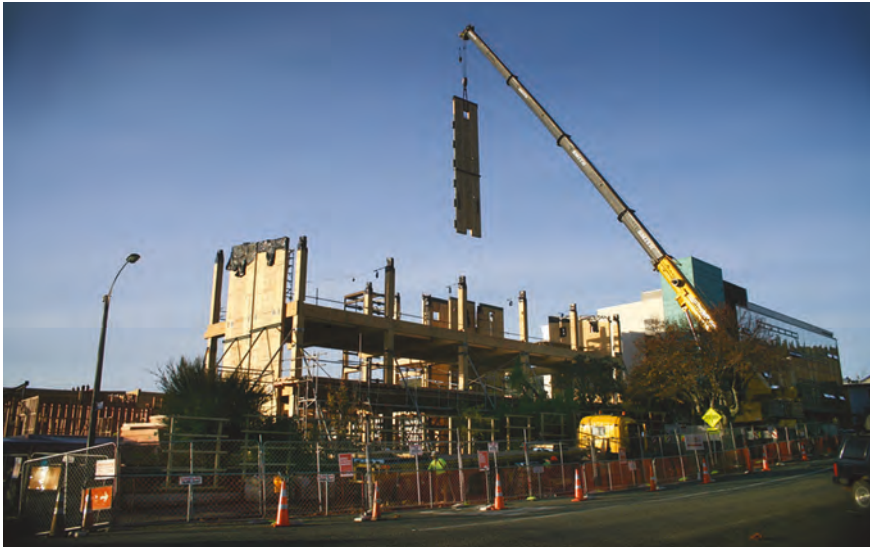
NMIT Arts & Media Building innovative post-tensioned timber rocking panel installation.
