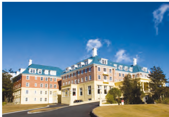
Chateau Tongariro modular extension and final construction.
