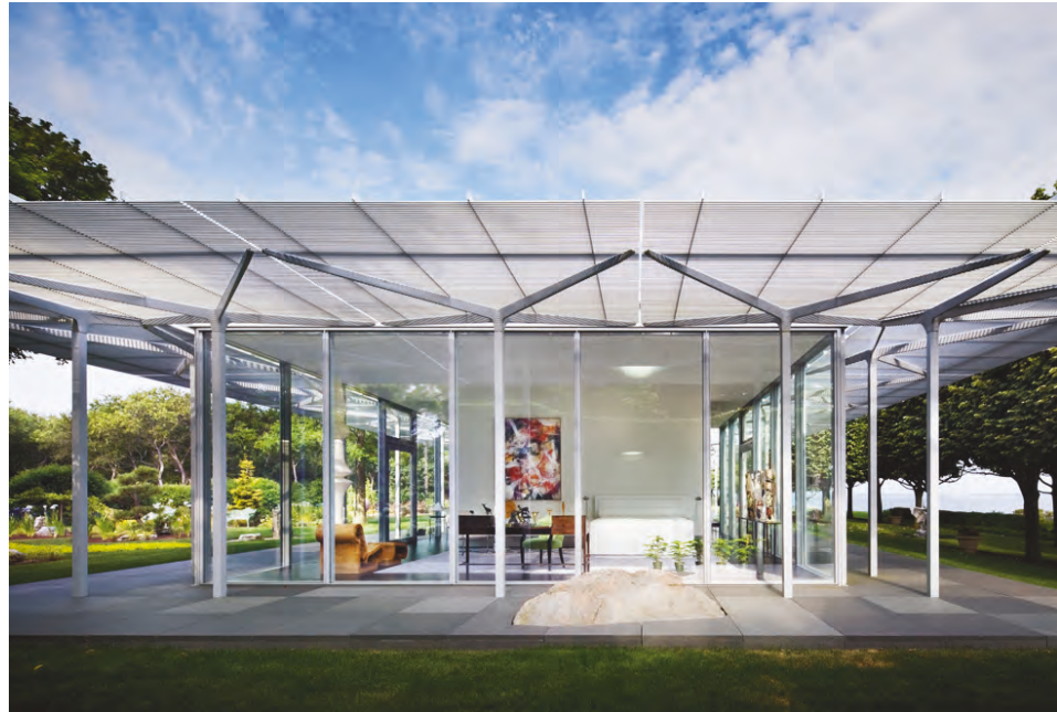
Fisher Island House by Thomas Phifer and Partners. A light modular steel and glass pavilion with major components built off site.
