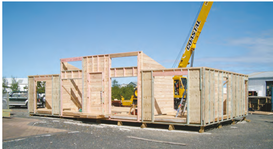
Touchwood wall panel assembly and wall panel assembly completed.
