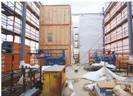
Modules stacked three high at site in Auckland.
