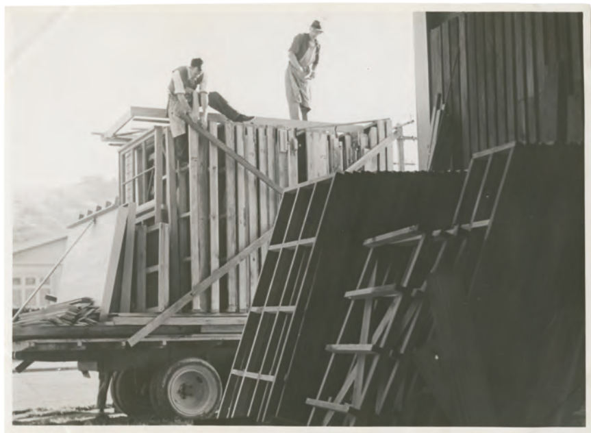
Returned soldiers headed by trained builders construct panelised state houses in the 1940s.
