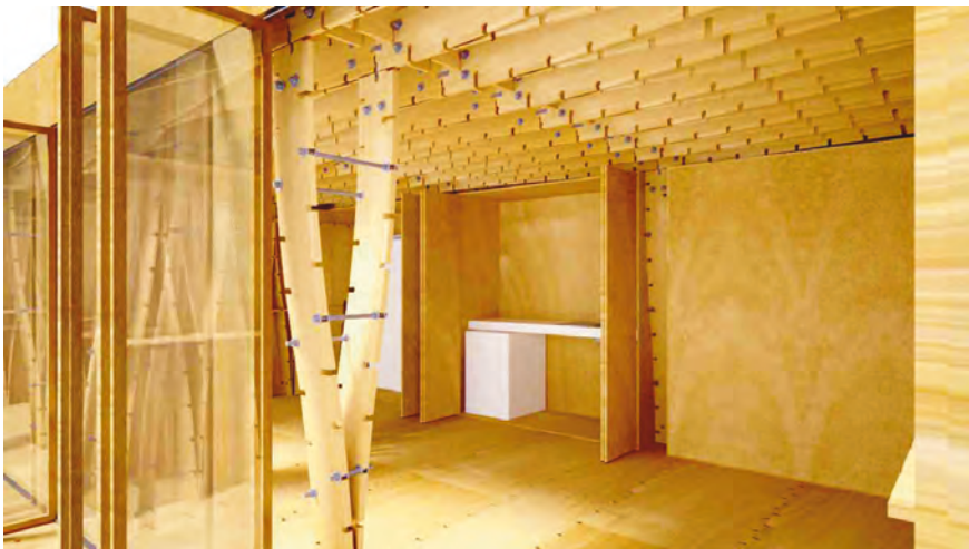
ABOVE: Massey CoCA by Athfield Architects interior with LVL beams and CNC router cut ceiling carving panels by Jacob Scott.
