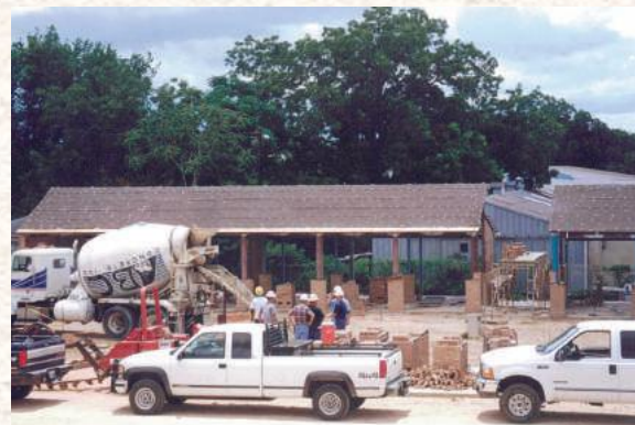
Plaza Saltillo under construction, 1999
