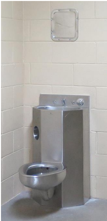
Figure 7 Image of combination toilet-sink facility used for going to the bathroom, brushing teeth, grooming, and obtaining hot water for preparing ramen noodles from the commissary. Image captured and cropped from Kripa and Mueller's article in The Architects Newspaper . Images were reportedly supplied by the agency.
