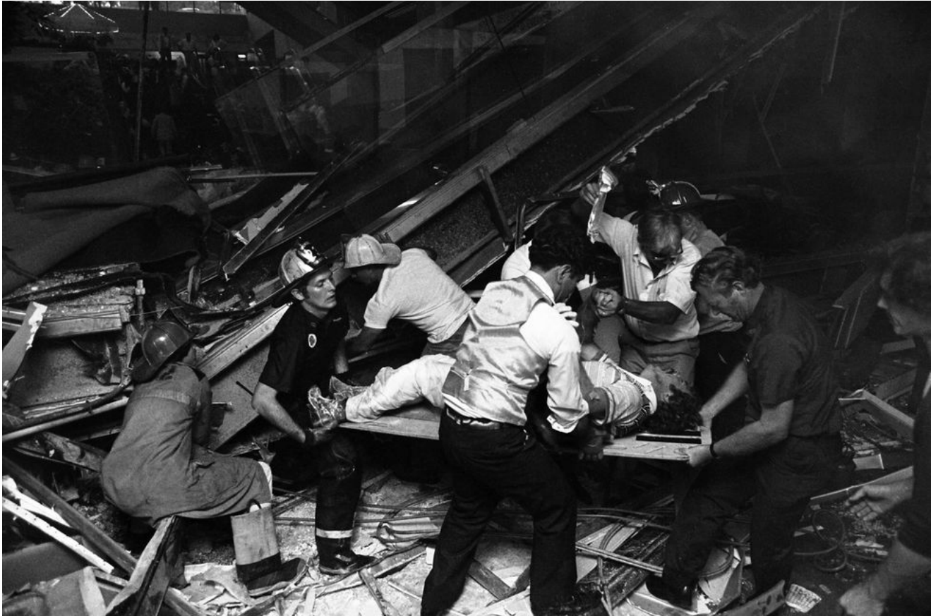
Firefighters rescue people from under a collapsed walkway. Bettmann/Getty Images
