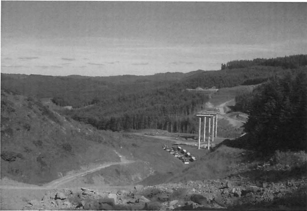
Fig. 2. View of road cut and bridge construction (Oregon Department of Transportation 2005).
