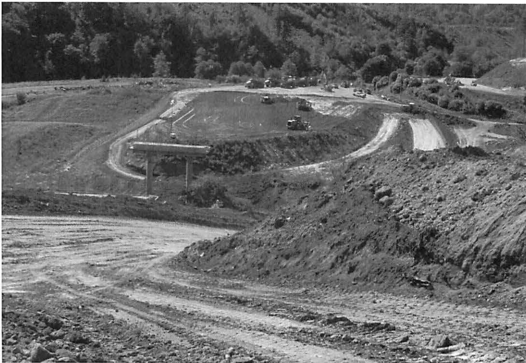
Fig. 3. View of road construction at Yaquina Meadows (Oregon Department of Transportation 2007).
