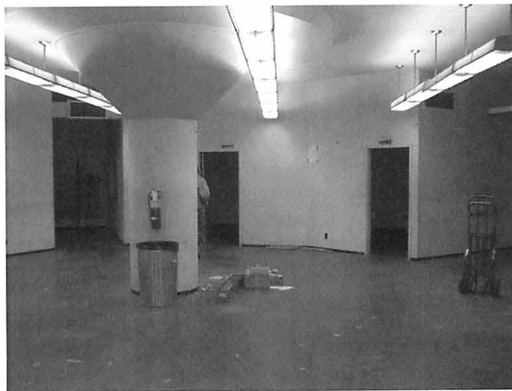
Fig. 5. Activity area surrounding the central pillar supporting 18-in. concrete roof, 5 ft. of highway fill, and the south-bound lanes of I-5. Behind the pillar (left to right) are the escape tunnel hallway, administrative office, and emergency medical room. (Photo by Craig Holstine, WSDOT, 2010).
