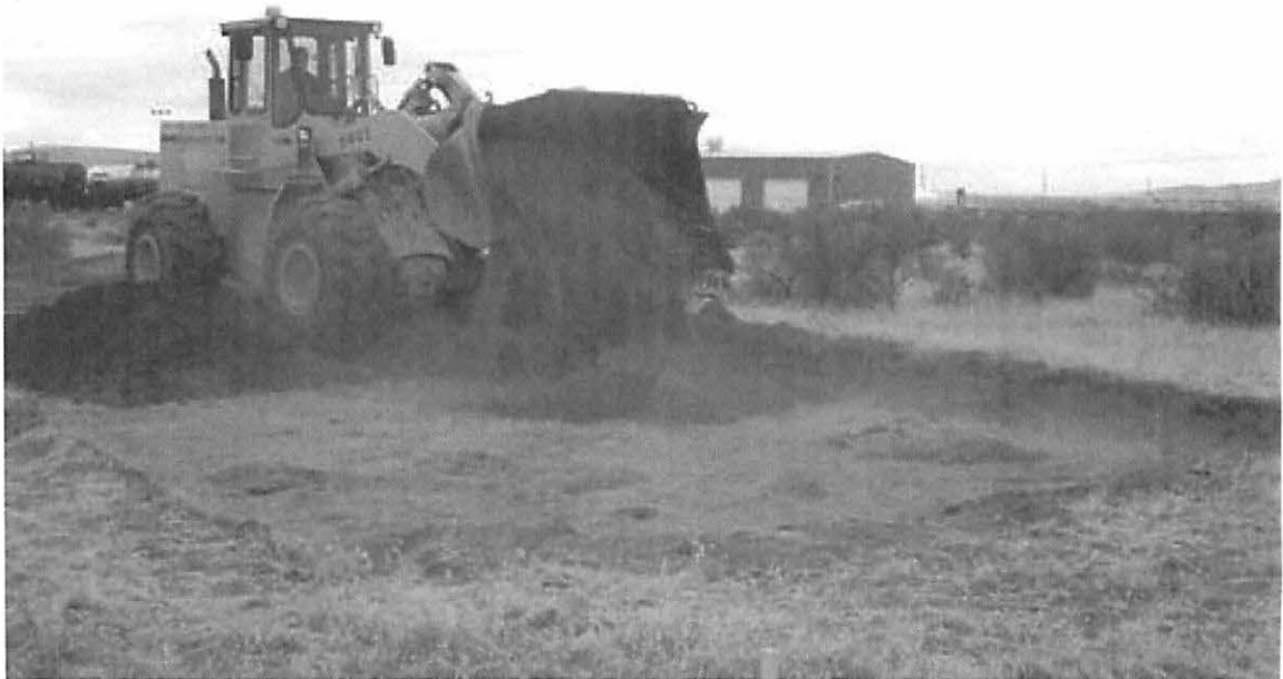
Fig. 3. Photograph showing the burying of simulated archaeological features in the Remote Target Test Bed using heavy equipment to carefully refill the trench with the original sandy material. September 2002.
