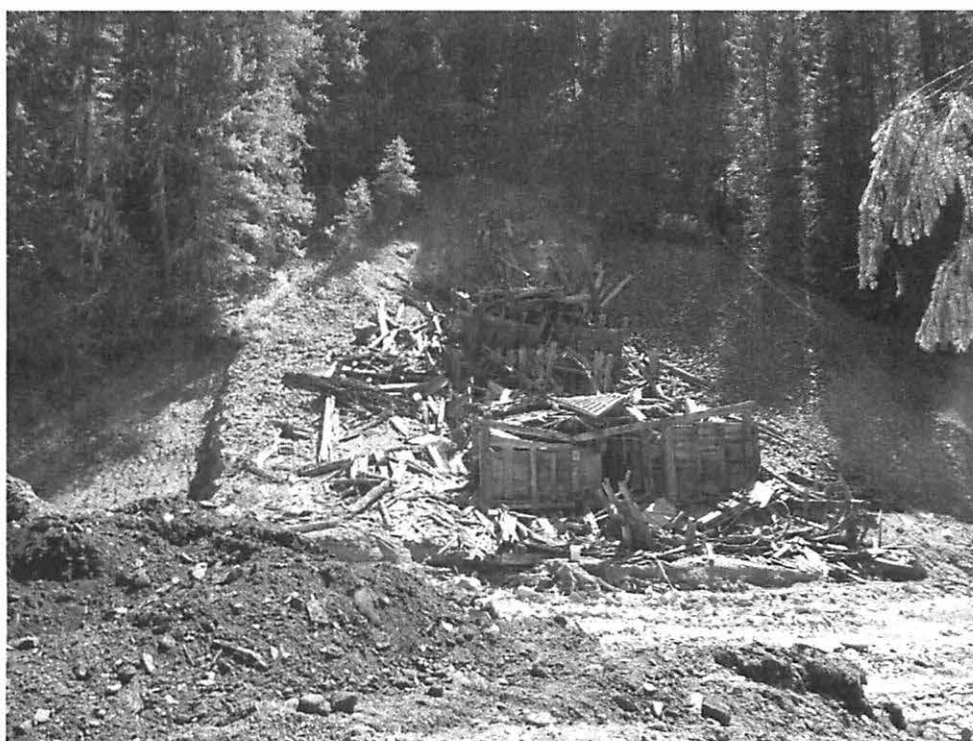
Fig 4. The Idora Mill site prior to removal: construction build-up in the foreground.
