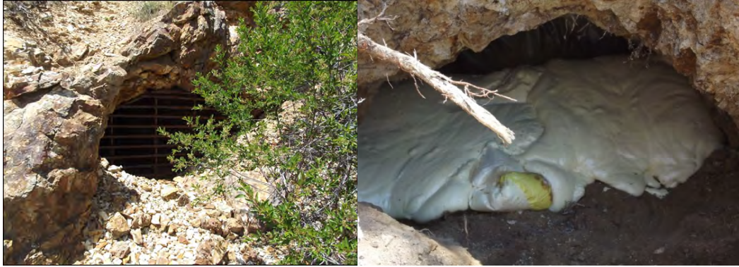
Figure 4: Gated adit on the left, adit closed by foam on the right.
