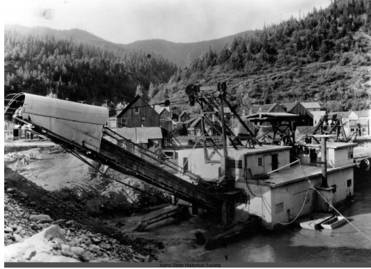
Figure 3: Dredge operated by the Yukon Gold Company near Murray, Idaho. Note sluices discharging fine tailings into the pond at the stern of the dredge. Larger rocks are being dumped on the large cobble pile by the tailings stacker. (Idaho, 2020f)
