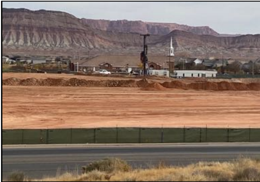
Figure 6: Photograph of New Temple Site from Field Survey
