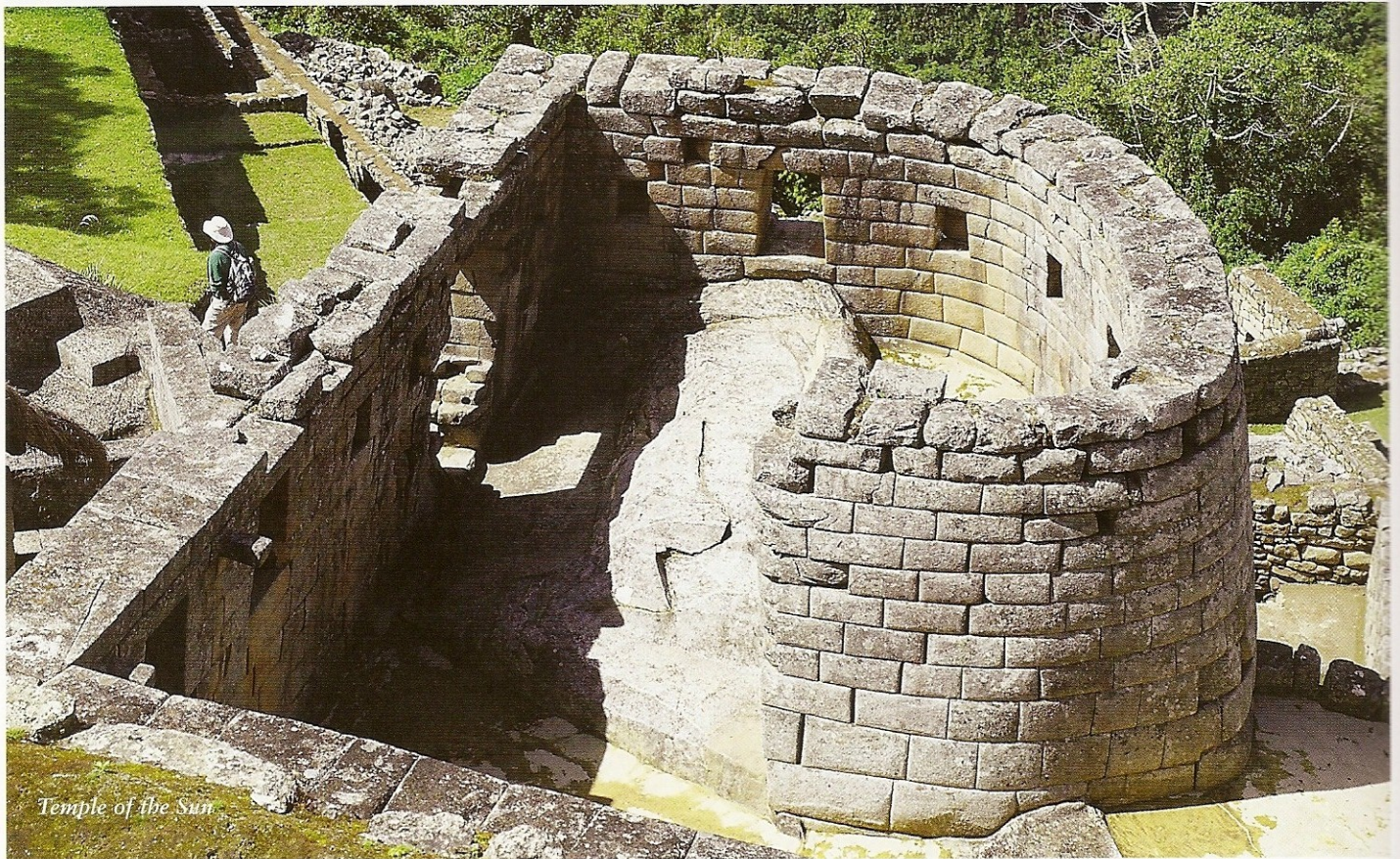
Expert masons often sliced stone blocks to fit flawlessly together without mortar.
