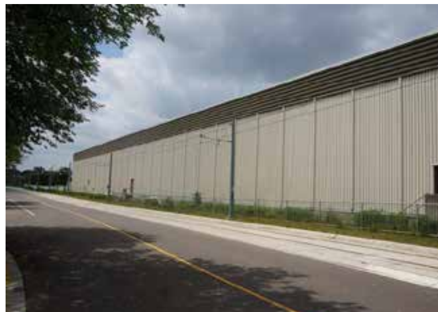
Borden Avenue South Streetscape
