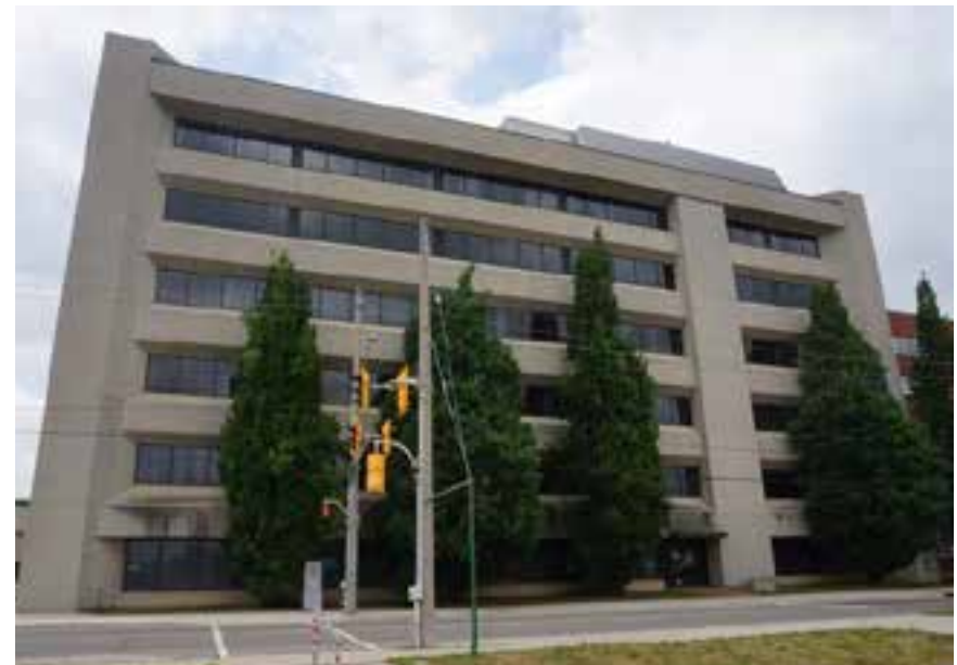
Existing Office on Courtland Avenue East
