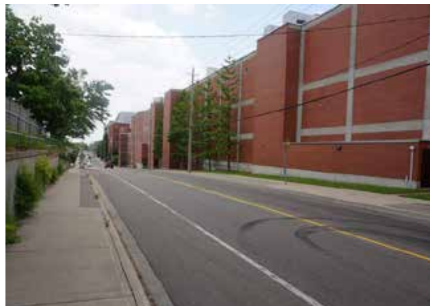
Courtland Avenue East Streetscape (pre-demolition)
