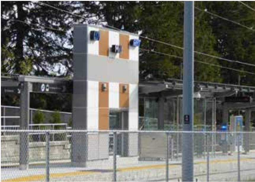
Mill Street ION LRT Station
