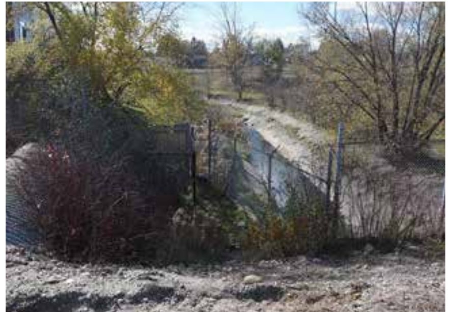
Schneider Creek Culvert south of CN Rail Corridor
