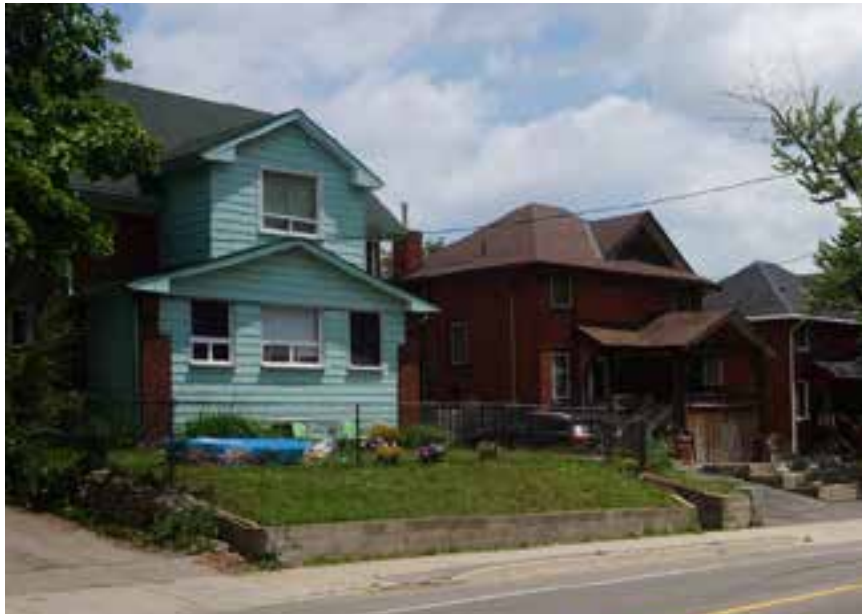
Single Detached Residential on Courtland Avenue East
