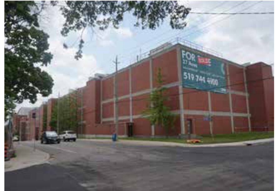
Former Plant Building on Courtland Avenue East
