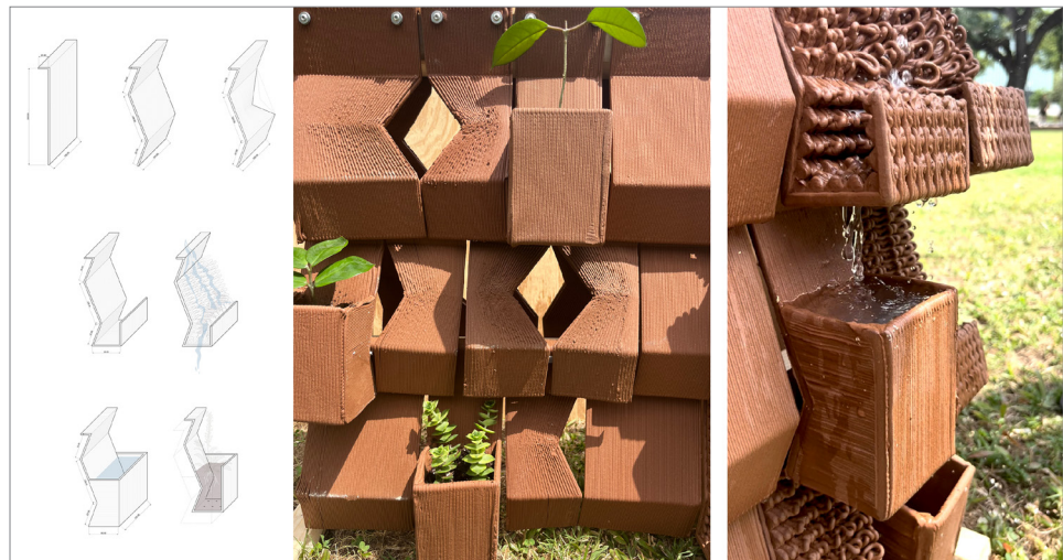
Figure 4. Collective Meander (S. Lindahl and D. Vorel). A simple shingle system includes multiple component types to serve different functions, such as providing apertures, serving as a gutter, and detaining stormwater (left). The full-scale mockup demonstrates the system's ability to accommodate a wide range of variation within its repetitive logic (center and right).
