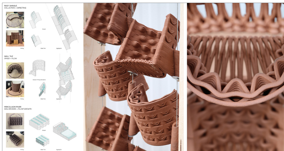
Figure 3. Ceramic Wetland (C. Kelley and S. Vladimir). Three types of ceramic modules (left) are designed to delay the flow of stormwater before it reaches the ground. The wall modules (center and right) integrate dense layers and scoops to detain water within the facade
