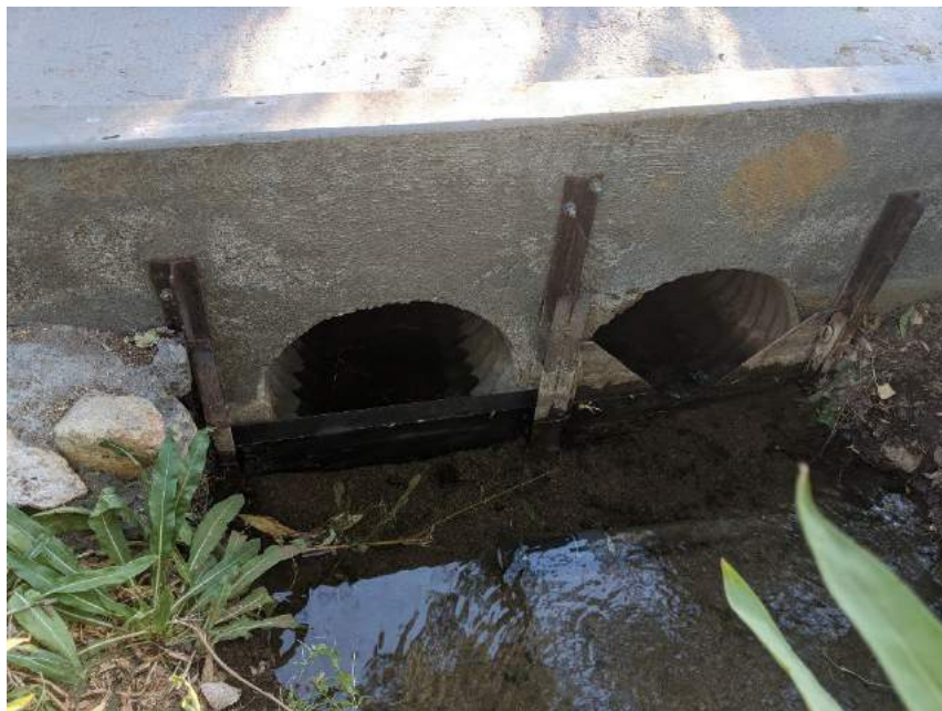
FIGURE 5. REHABILITATED SHARP CRESTED WEIR ON THE LEFT CULVERT OPENING.
