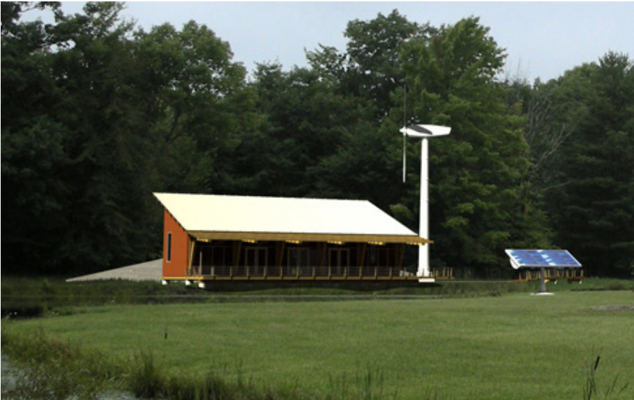
Above: Power generation and water heating from the roof provide over 80% of the energy requirements for Beaumont Environmental Education Center
