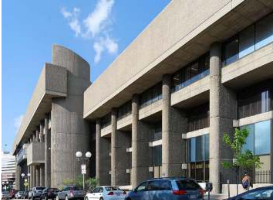
1. Hurley Building, west elevation, view northeast
