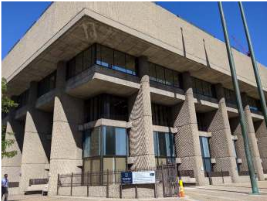
2. Hurley Building, west elevation (left) and south elevation (right), view northeast
