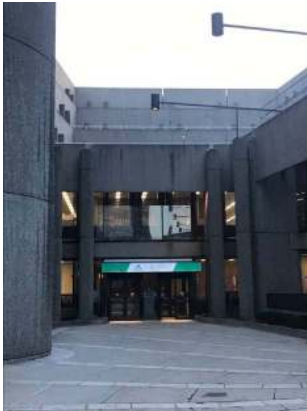
14. Hurley Building, interior courtyard entrance, view southwest
