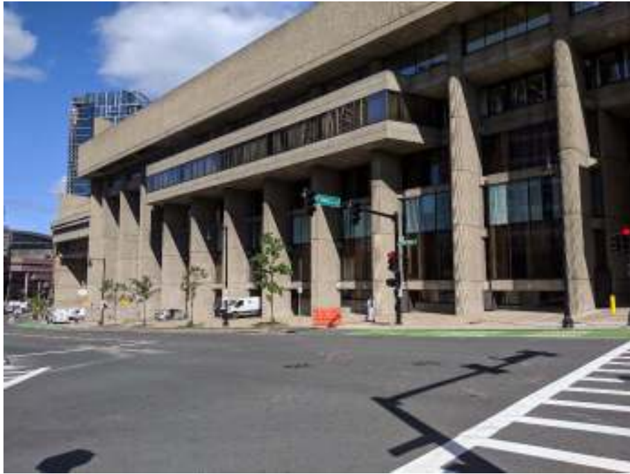
7. Hurley Building, west elevation, view northeast
