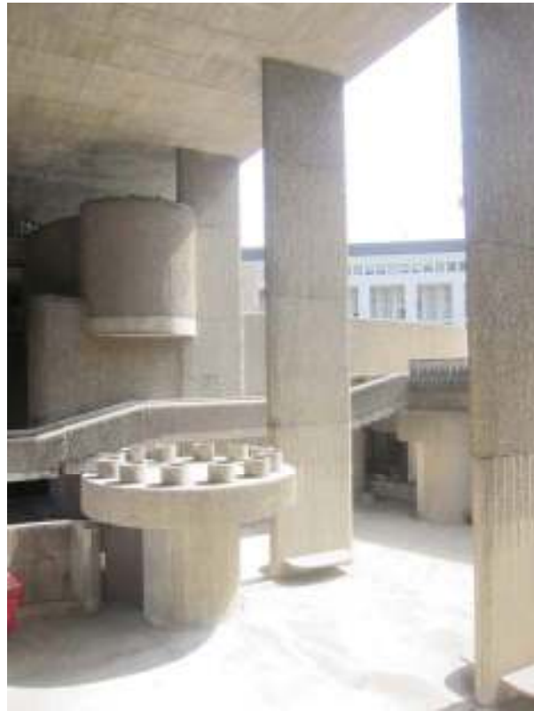
22. Recessed enclosure, Lindemann Center, view southeast
