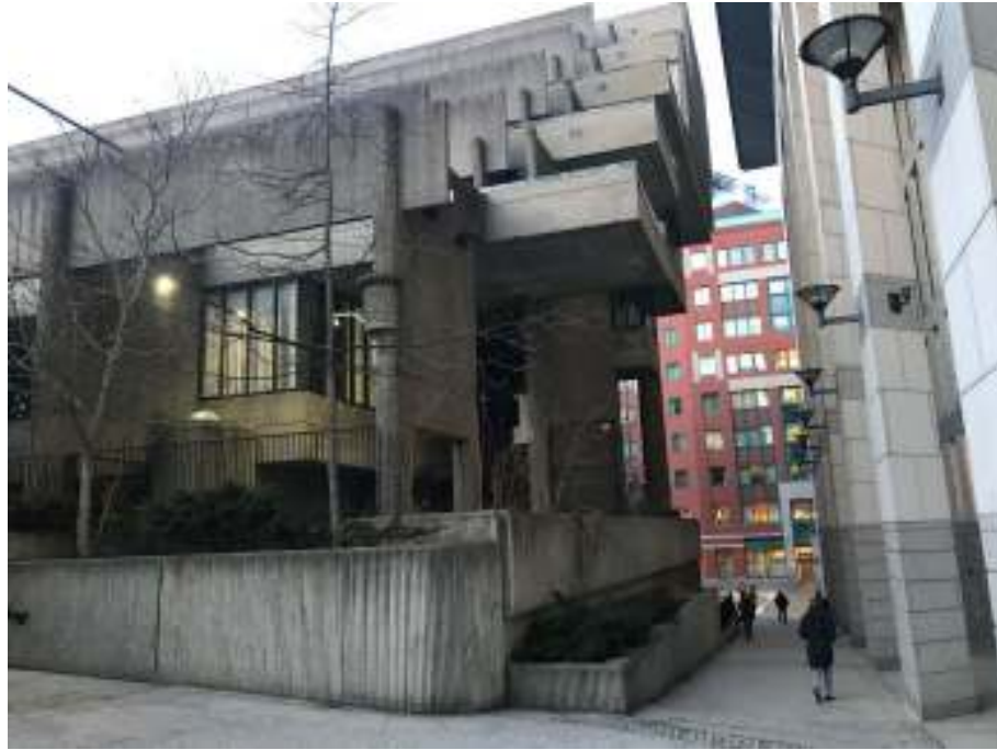
21. Interior courtyard, view north toward Lindemann Center and pedestrian passage between Lindemann Center and Brooke Courthouse
