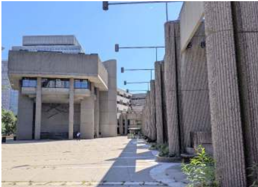
20. Interior courtyard, Hurley Building, view south
