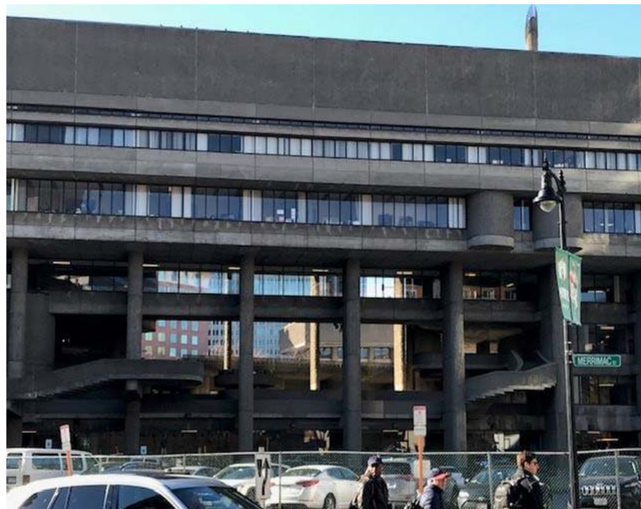
24. Northwest elevation of the Lindemann Center, view southeast
