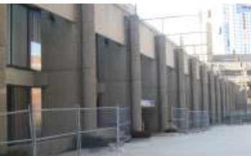
Figure 4.9: Courtyard facade at H7- oblique prior to new steel balustrades.
