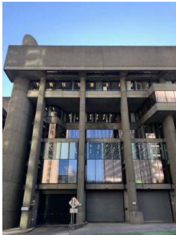
6. Hurley Building, west elevation detail, view east
