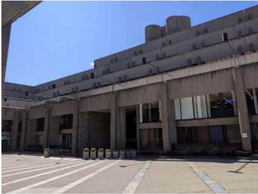
17. Interior courtyard, Hurley Building, view southwest
