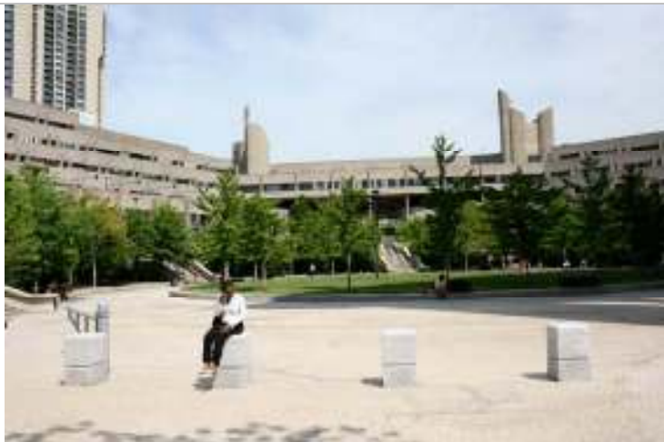
Courtyard - View to northwest
