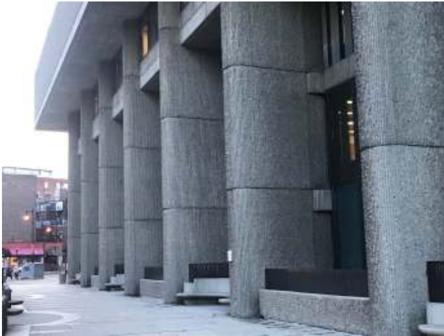
8. Hurley Building, east elevation, view southwest
