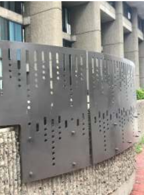
Figure 4.1: 2019 Protection at Plaza light wells
