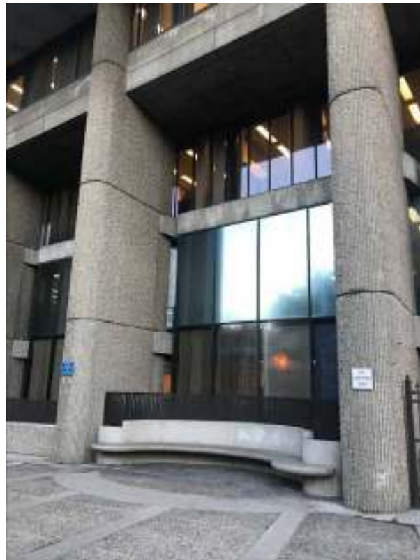
4. Hurley Building, west elevation detail, view east
