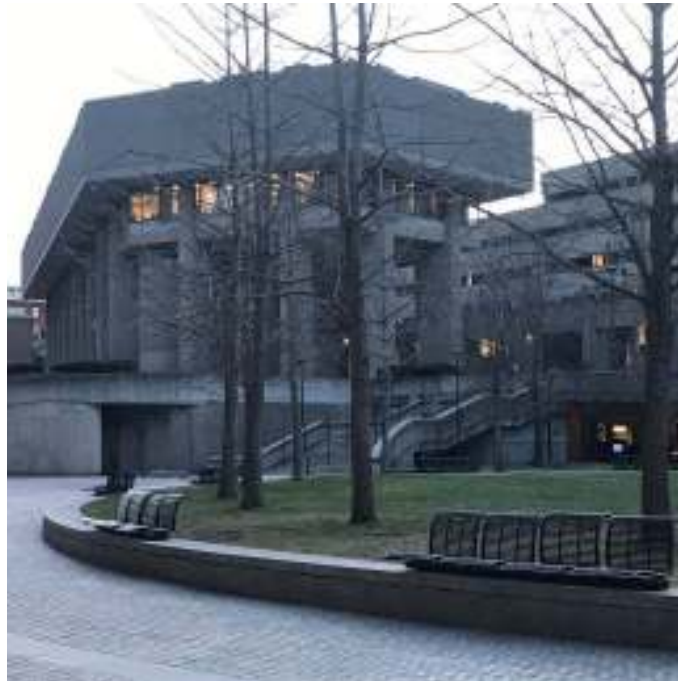
10. Hurley Building east elevation, view southwest
