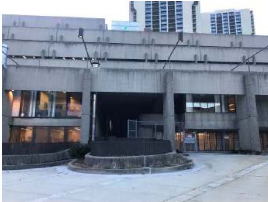
19. Interior courtyard, view west of party wall and passage between Hurley Building (left) and Lindemann Center (right)
