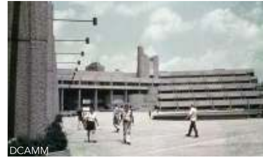
Figure 3.5: Interior courtyard showing stepped facade (L4/5).
