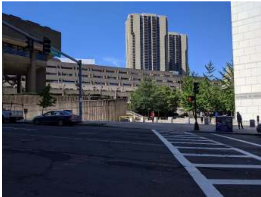
12. Interior courtyard, Hurley Building (left) and Lindemann Center (extreme right), view northwest
