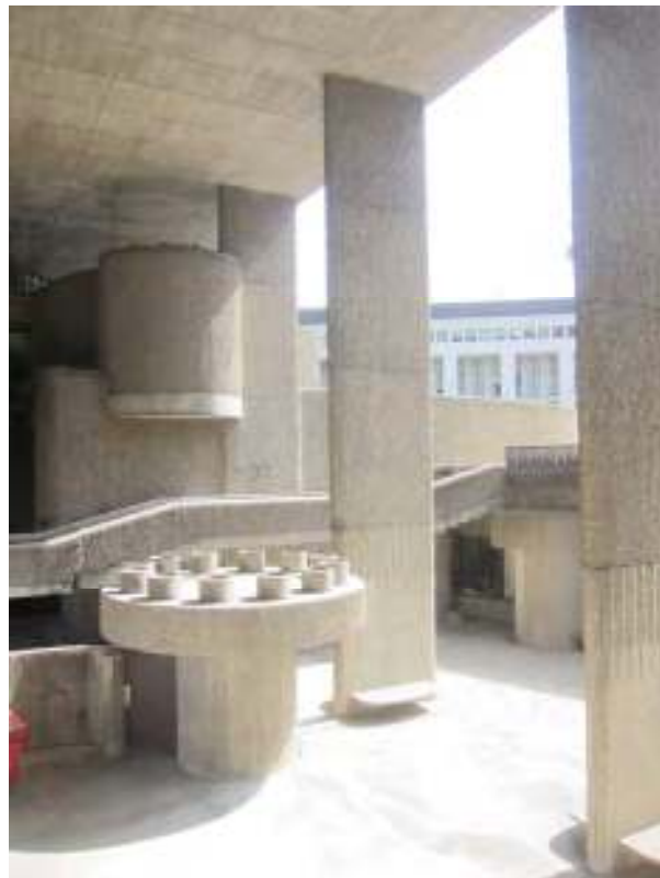
22. Recessed enclosure, Lindemann Center, view southeast
