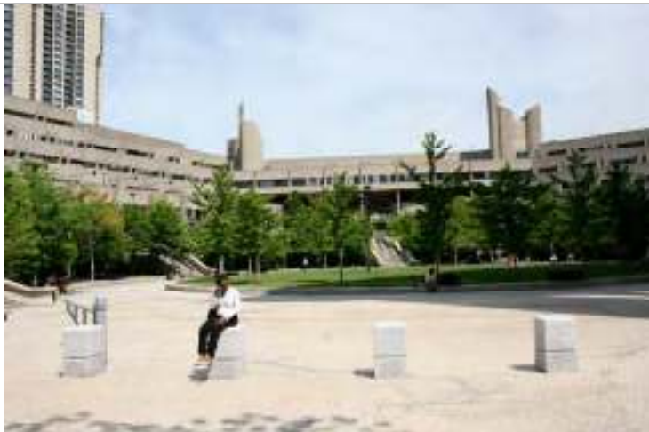
Courtyard - View to northwest
