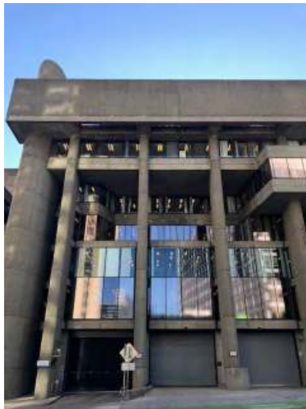
6. Hurley Building, west elevation detail, view east
