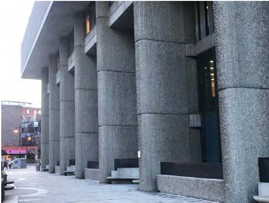
8. Hurley Building, east elevation, view southwest
