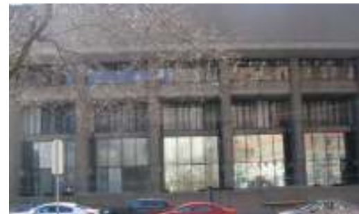
Figure 4.13: Reflective solar films on windows at H3 facade.
