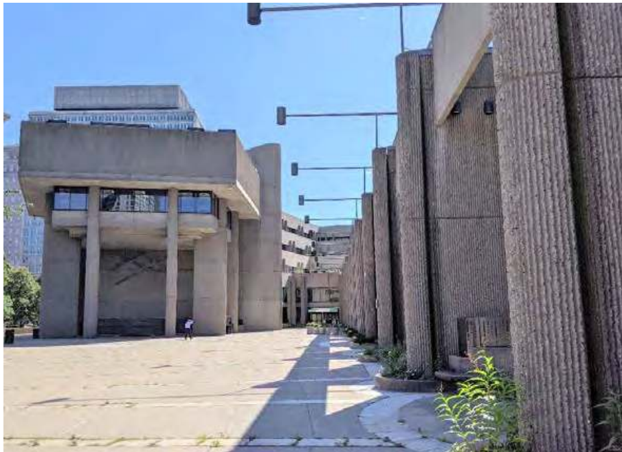
20. Interior courtyard, Hurley Building, view south
