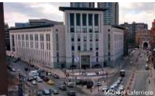
Figure 4.17: Intersection of Merrimac and New Chardon Streets in front of the Brooke Courthouse.
