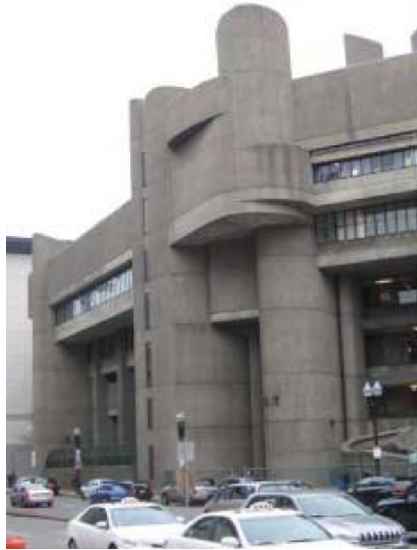
23. North (left) and northwest (right) elevations of Lindemann Center, view southeast
