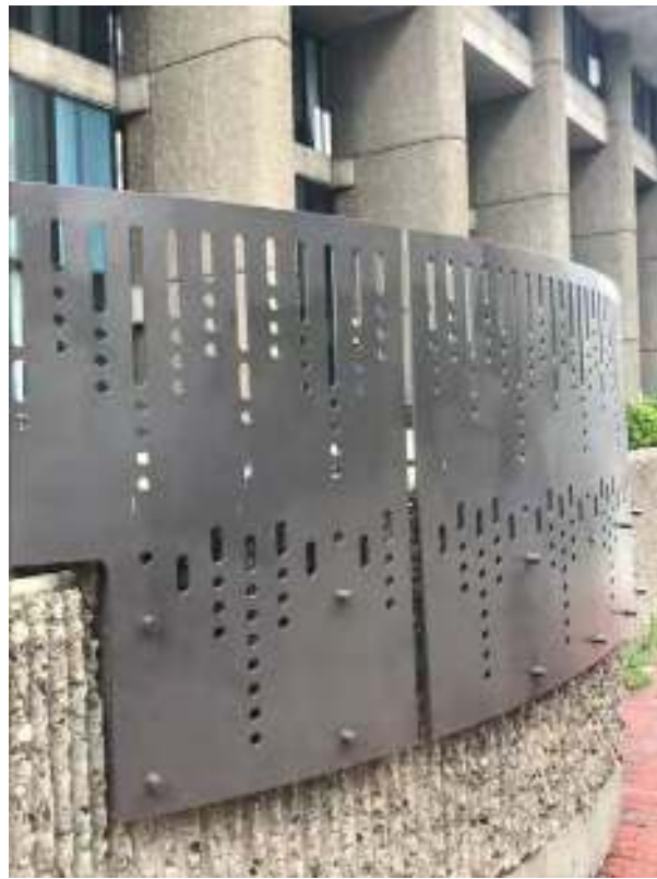
9. Hurley Building, east elevation detail, modern safety railing, view northwest
