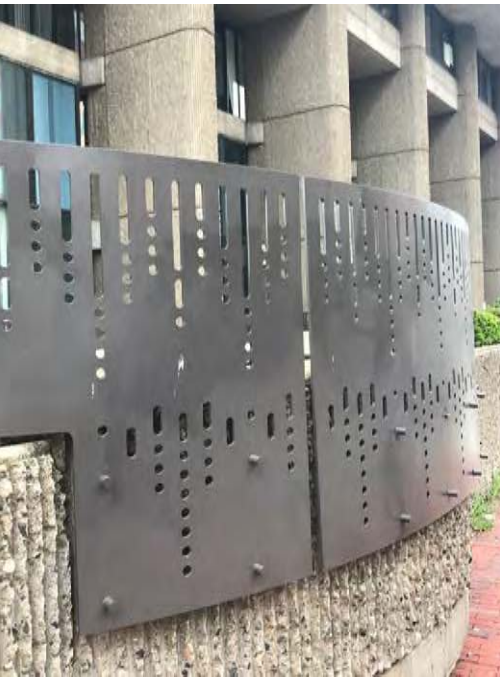
Figure 4.1: 2019 Protection at Plaza light wells
