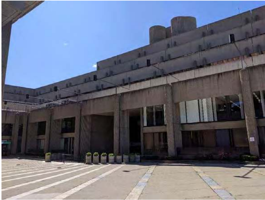
17. Interior courtyard, Hurley Building, view southwest
