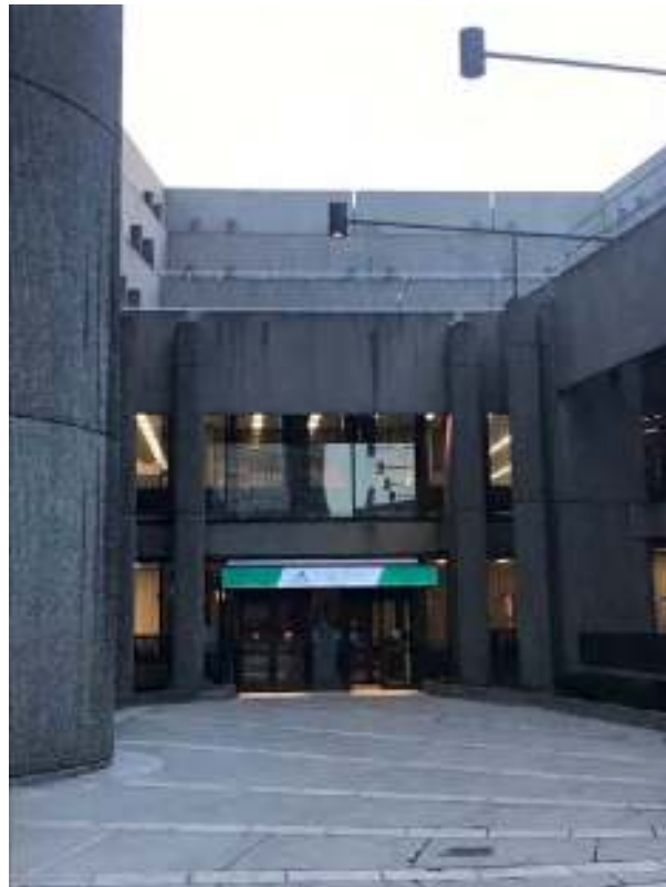
14. Hurley Building, interior courtyard entrance, view southwest
