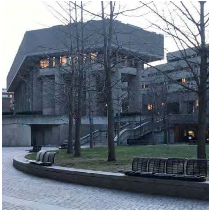
10. Hurley Building east elevation, view southwest
