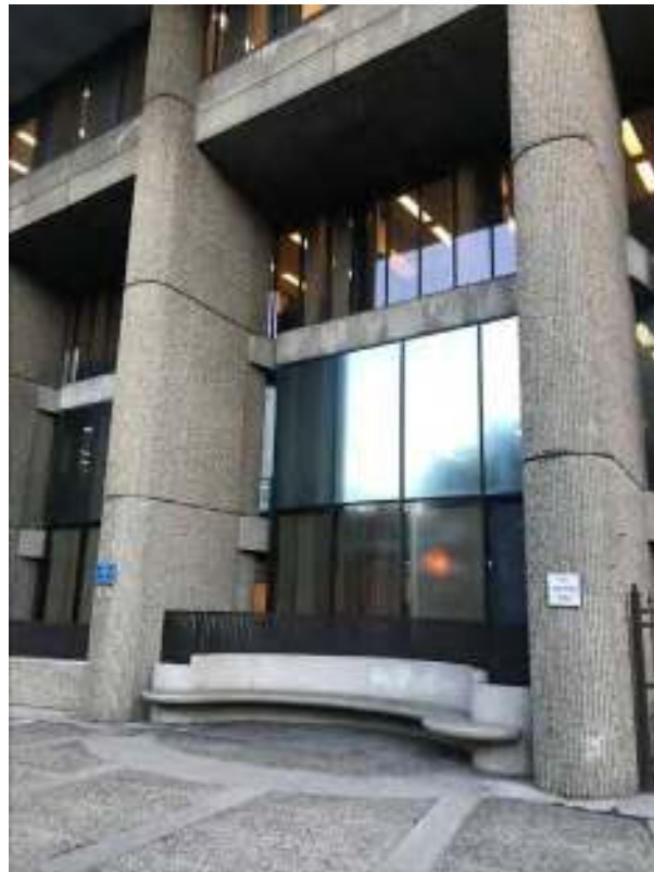
4. Hurley Building, west elevation detail, view east
