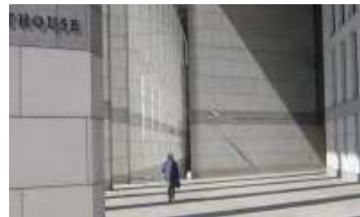
Figure 4.6: Courtyard arcade of the Brooke Courthouse.
