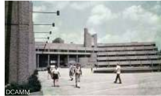
Figure 3.5: Interior courtyard showing stepped facade (L4/5).
