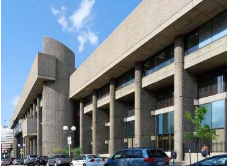
1. Hurley Building, west elevation, view northeast
