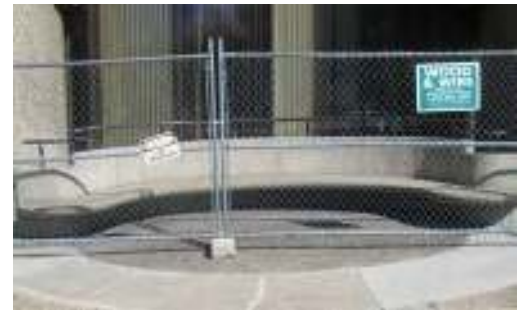
Figure 4.12: Fenced-off concrete bench at H1 prior to new steel balustrades.
