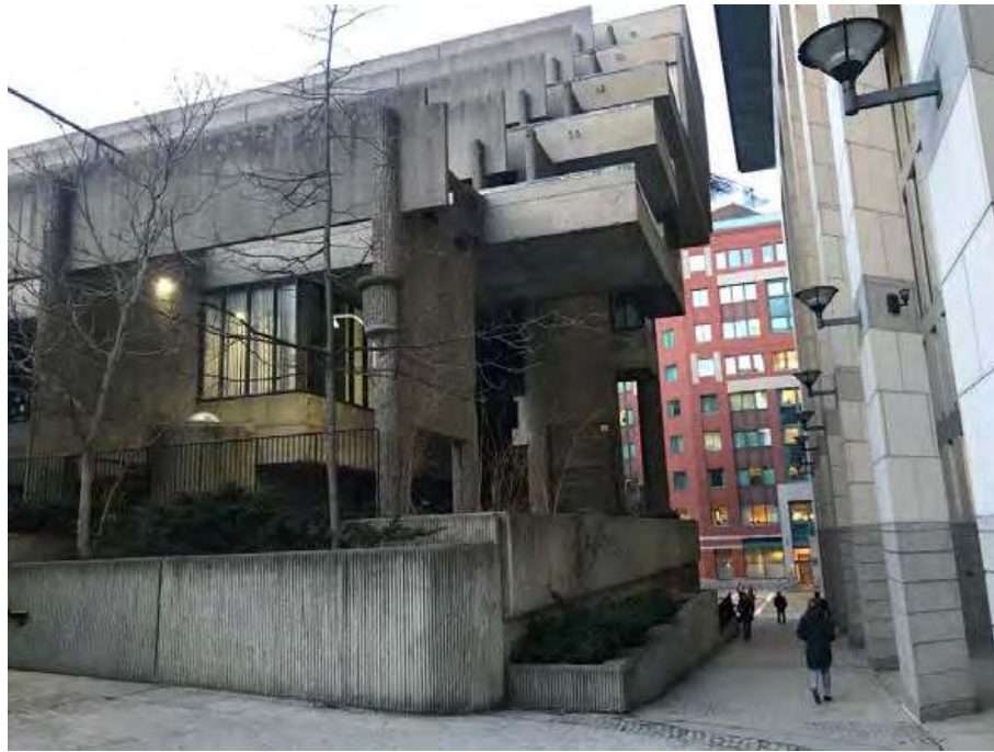
21. Interior courtyard, view north toward Lindemann Center and pedestrian passage between Lindemann Center and Brooke Courthouse
