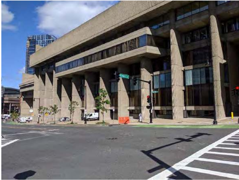
7. Hurley Building, west elevation, view northeast
