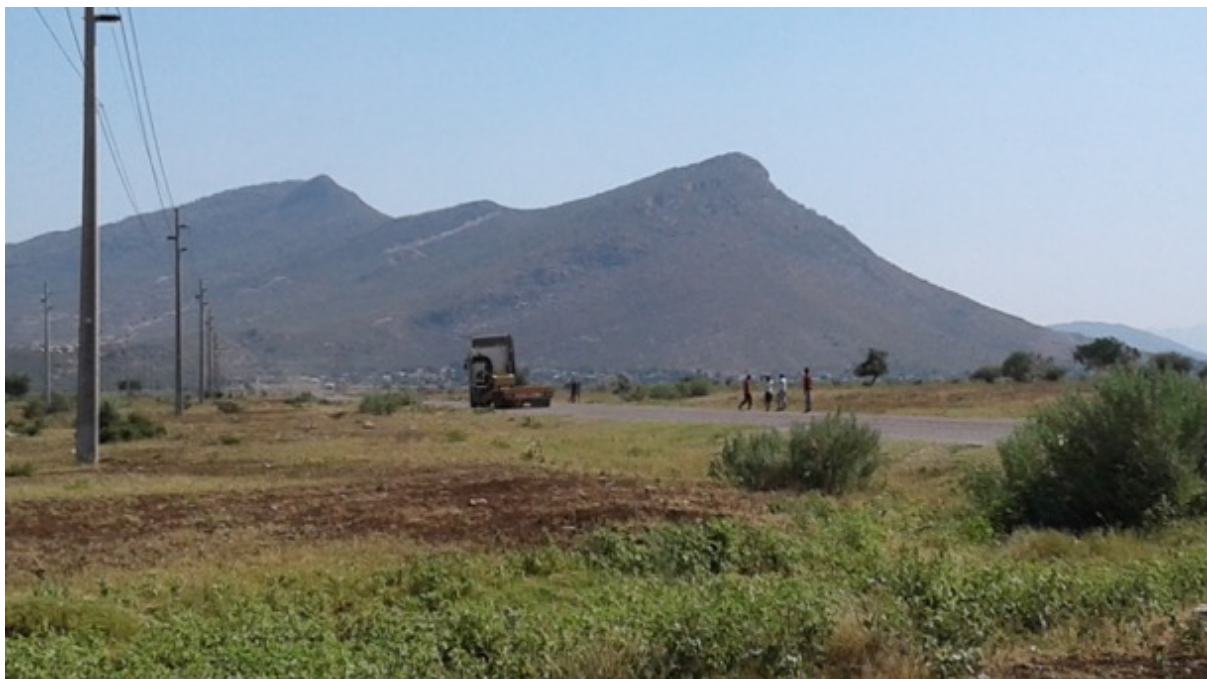
Power lines and tarred road constructed on arable land
