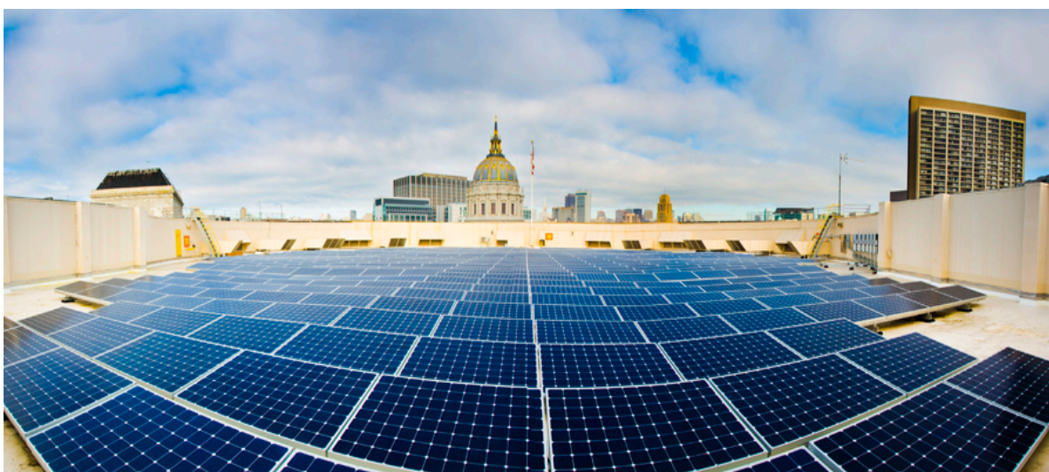
Photo 7: Davies Symphony Hall Solar Panel Installation
