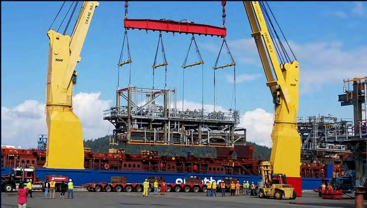
Andeavor Refinery Modules T-Bailey Pipe Canadian Coast Guard Vessels
