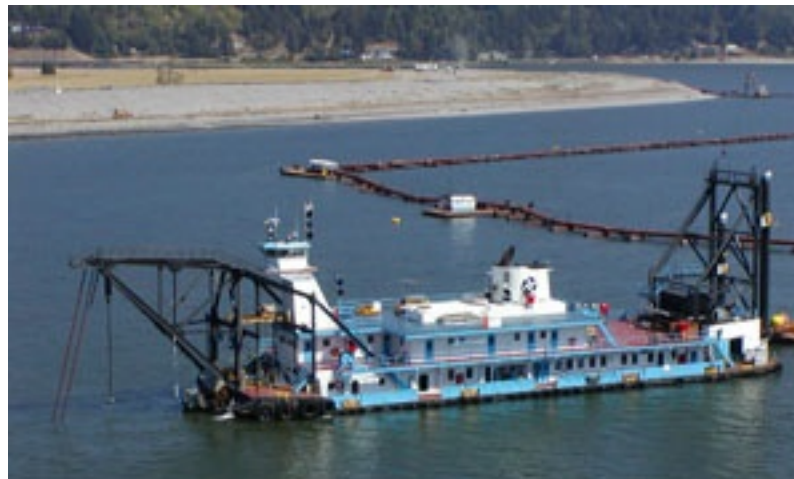
Port of Portland dredge Oregon
