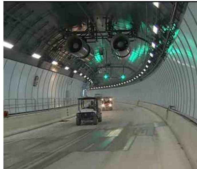
Port of Miami Tunnel was designed to withstand 10 feet of sea-level rise
