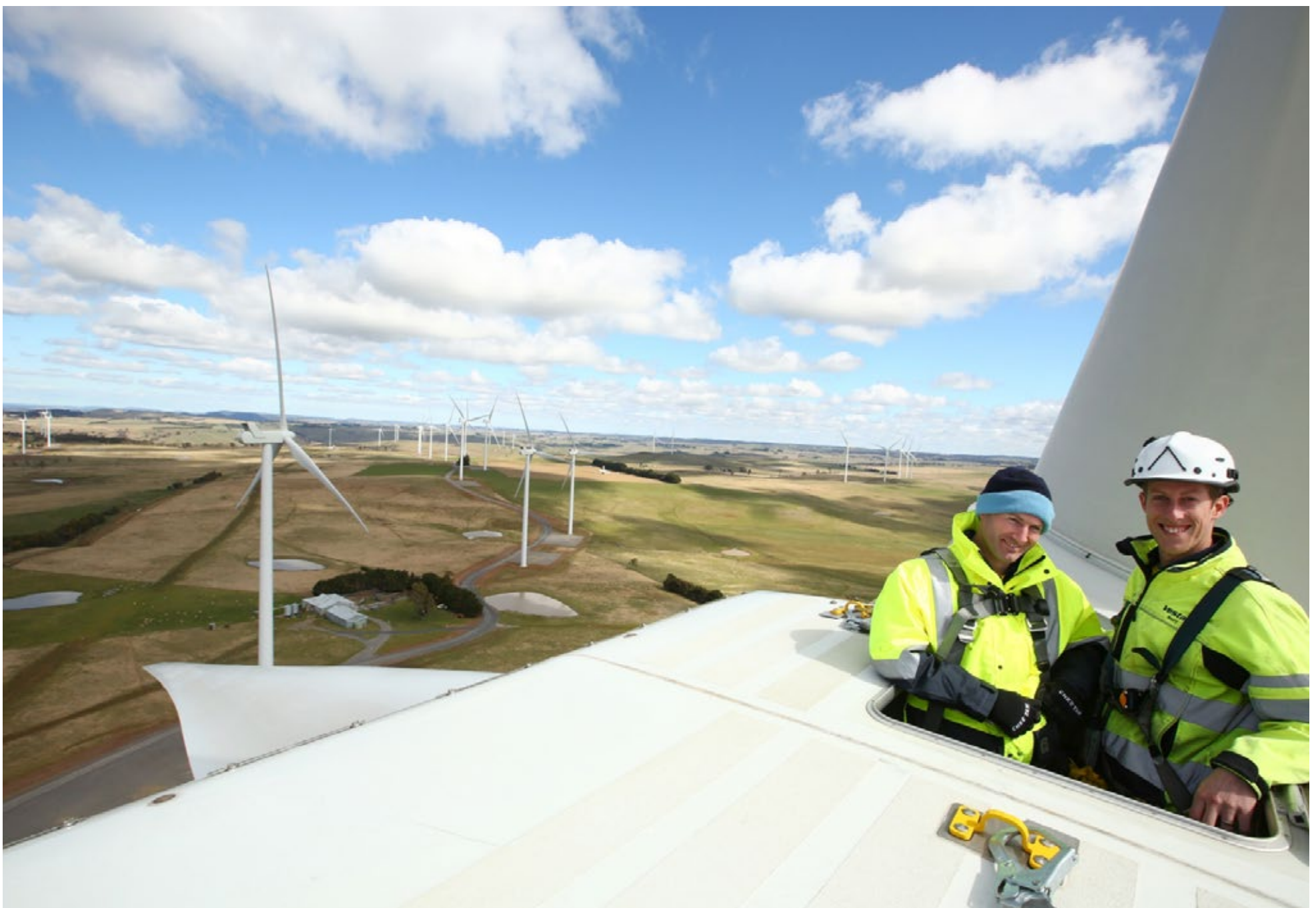
Turbine engineers commissioning a machine at Taralga Wind Farm. Photo by CWP Renewables.
