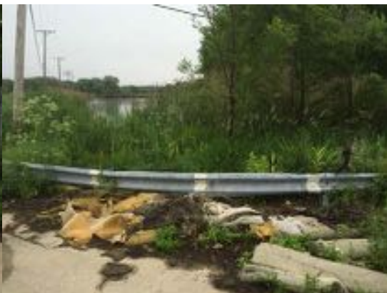
Fly dumping along site access road at 134 th Street
