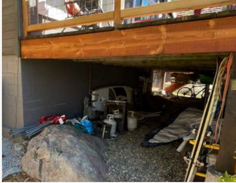
Before and After: Combustible stored under stored under deck cleaned up to remove ignition materials & propane tanks.
