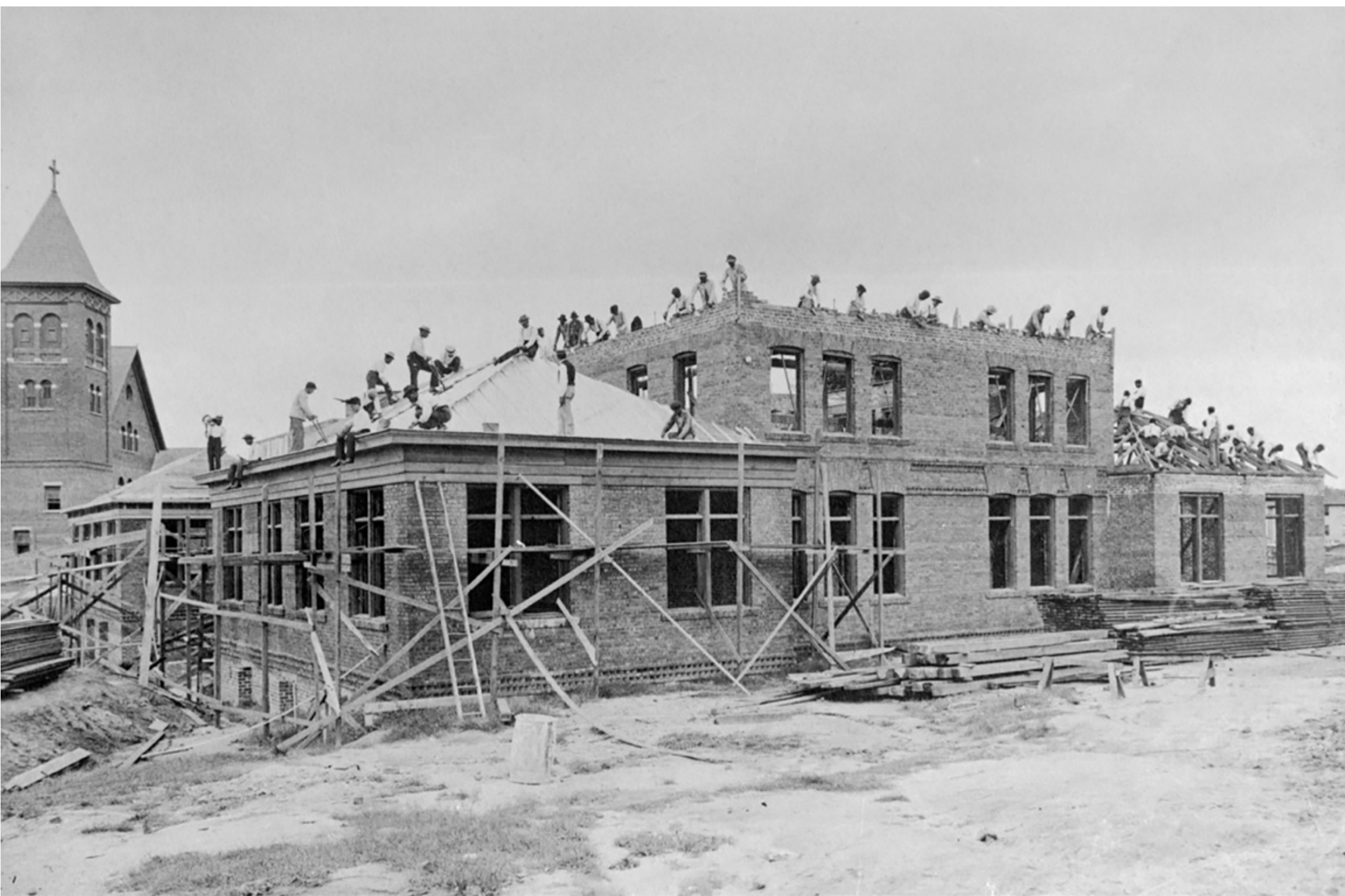
TUSKEGEE INSTITUTE STUDENTS WORKING ON NEW BUILDING. BETTMANN/GETTY IMAGES
