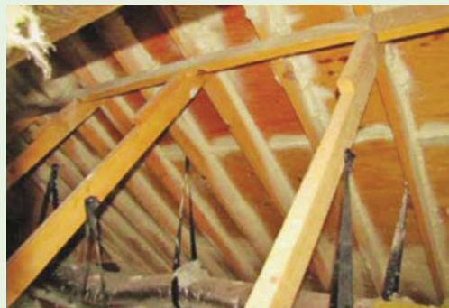
Figure 4-5. Spray polyurethane foam is used to add strength between the rafters and the plywood sheathing. This method can be used to strengthen existing roofs and may negate the need to replace older roofs. It can also be used where fasteners are missing or at the corners of hip style roofs or the ends of gable end roofs, which are especially susceptible to wind forces. See FEMA publication numbers P-499 and P-804. Image courtesy of FEMA
