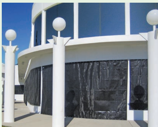
Figure 4-17. Polyethylene basketweave fabric windscreens deployed directly over ground floor windows of a coastal home. Image courtesy of Roll-a-way
