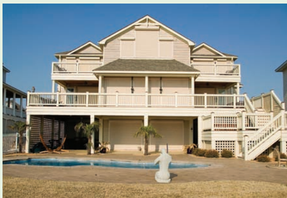
Figure 4-11. Coastal home protected with roll-down shutters on all windows and doors. The shutter is held in place by vertical guide tracks and can be deployed manually or with an integrated electric motor. Image courtesy of QMI, Inc.
