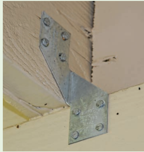
Figure 4-9. This is an example of retrofitting an existing house originally built without hurricane clips. The popular H3 clip is used here; four nails attach the clip to the roof (truss-rafter) and four more nails attach to the wall or top plate below. For a retrofit, the clips are exposed on the outside of the house; therefore, both the clip and fasteners should be corrosion-resistant and painted to blend with the exterior of the house. With the correct clip and nails, you could perform the work or, if you prefer, hire a licensed contractor. Image courtesy of Dennis Hwang
