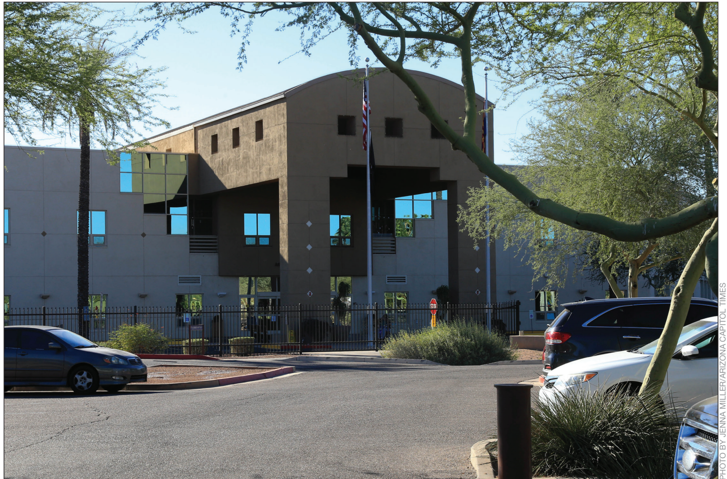
The Arizona State Veterans Home in Phoenix, near Indian School Road and Third Street, is a 200-bed nursing care facility.
