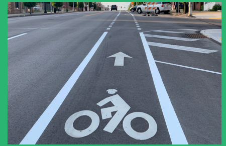
Newly installed bike lines along 7th Avenue in Beaver Falls
