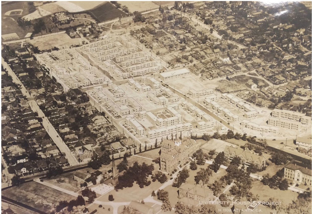
Construction of University Homes, Black residential enclave, Atlanta, GA, c. 1936. Charles F. Palmer papers, Box 167, Folder 10 (Atlanta, Georgia: Emory University Stuart A. Rose Manuscript, Archives, and Rare Book Library).
