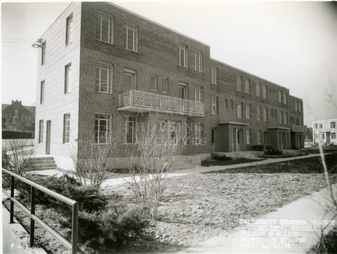
University Homes two-story apartment type under construction, Atlanta, GA, 1936. University Homes Records, photograph UNIV2013_img_01711 (Atlanta, Georgia: Atlanta Housing Archives, The Housing Authority of the City of Atlanta).
