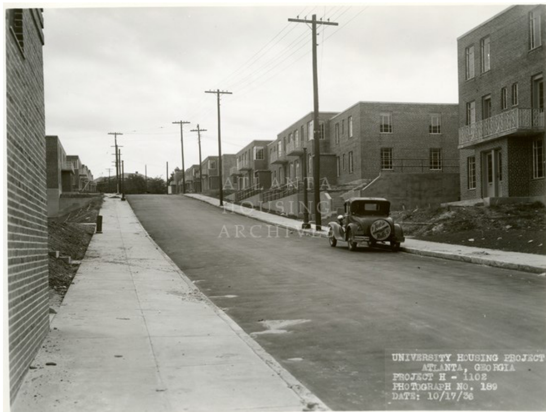
University Homes street view under construction, Atlanta, GA, 1936. University Homes Records, photograph UNIV2013_img_01666 (Atlanta, Georgia: Atlanta Housing Archives, The Housing Authority of the City of Atlanta).
