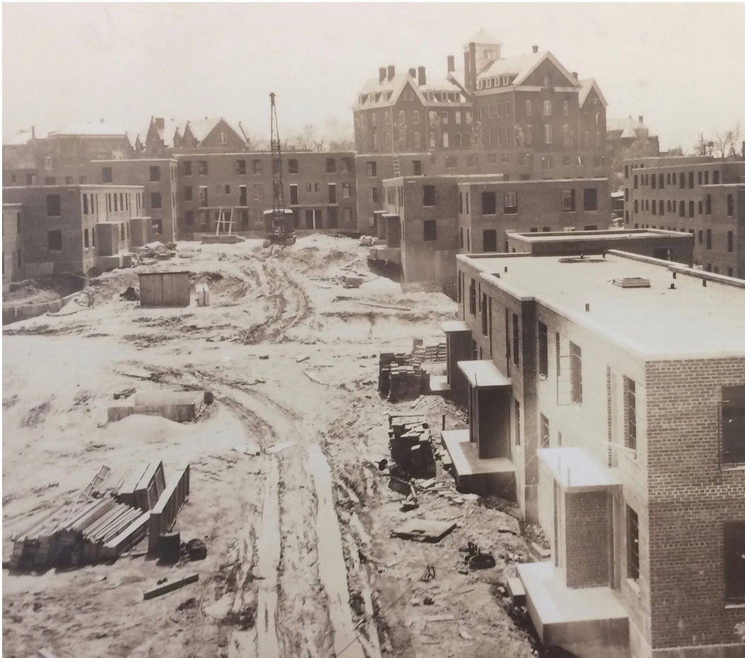
Construction of University Homes, with Spelman College in the background, Atlanta, GA, c. 1936. PWA Housing Division photograph, Charles F. Palmer papers, Box 167, Folder 10 (Atlanta, Georgia: Emory University Stuart A. Rose Manuscript, Archives, and Rare Book Library).
