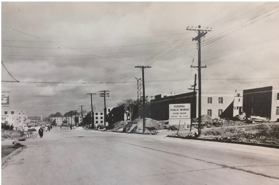
Techwood Homes under construction with PWA Housing Division sign in foreground, c. 1935. Charles F. Palmer papers, Box 167, Folder 8 (Atlanta, Georgia: Emory University Stuart A. Rose Manuscript, Archives, and Rare Book Library).
