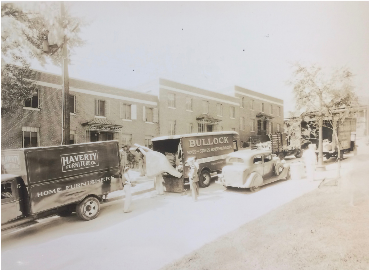
Families moving into row houses on Merritts Avenue, Building 3, Group 109, official opening Techwood Homes, Sept. 1, 1936. Charles F. Palmer papers, Box 167, Folder 9 (Atlanta, Georgia: Emory University Stuart A. Rose Manuscript, Archives, and Rare Book Library).
