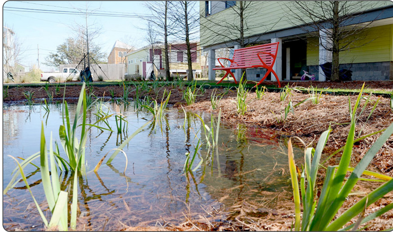
Photo: Conversion of a vacant lot into a stormwater management device (New Orleans Redevelopment Authority).
