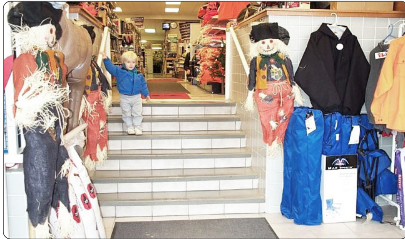
Photos: Floodproofed vestibule with elevated primary livable space in Darlington, Wisconsin (U.S. Army Corps of Engineers).
