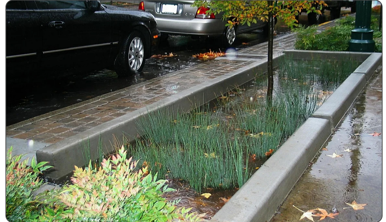
Photo: Landscaped planters cleaning and absorbing stormwater along the street (Kevin Robert Perry / Urban Rain Design).
