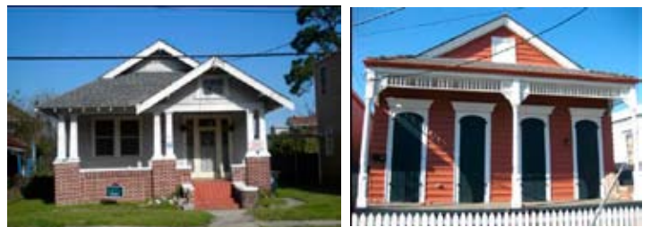
217 S. Tonti and 2422 Palmyra St are both renovated houses in the footprint of the medical district. ( www.savemidcityhouses.com )
