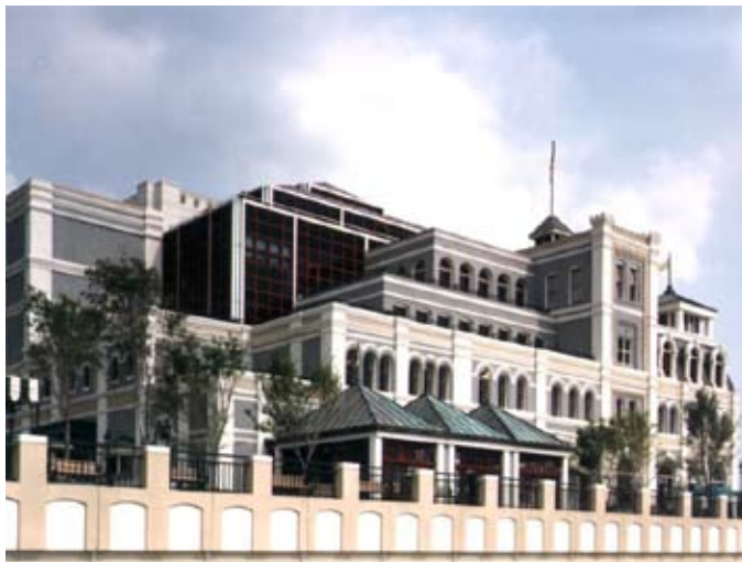
Jackson Brewery Back - contemporary materials and details facing riverside.
