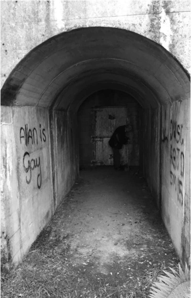
Inchindown oil tank entrance, Scotland
